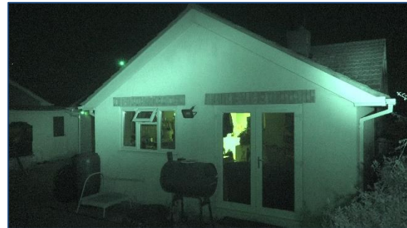
North and west gable – second survey
