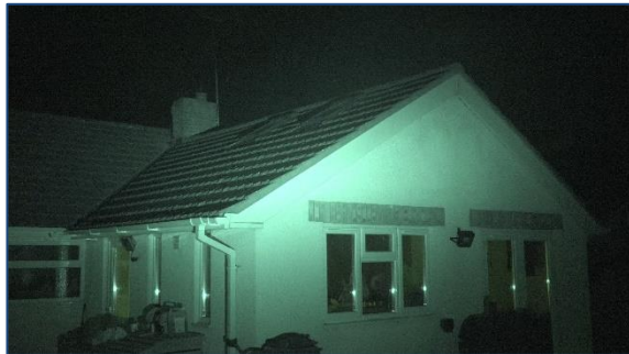
North gable – first survey
