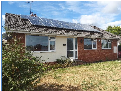
Building exterior – south elevation
