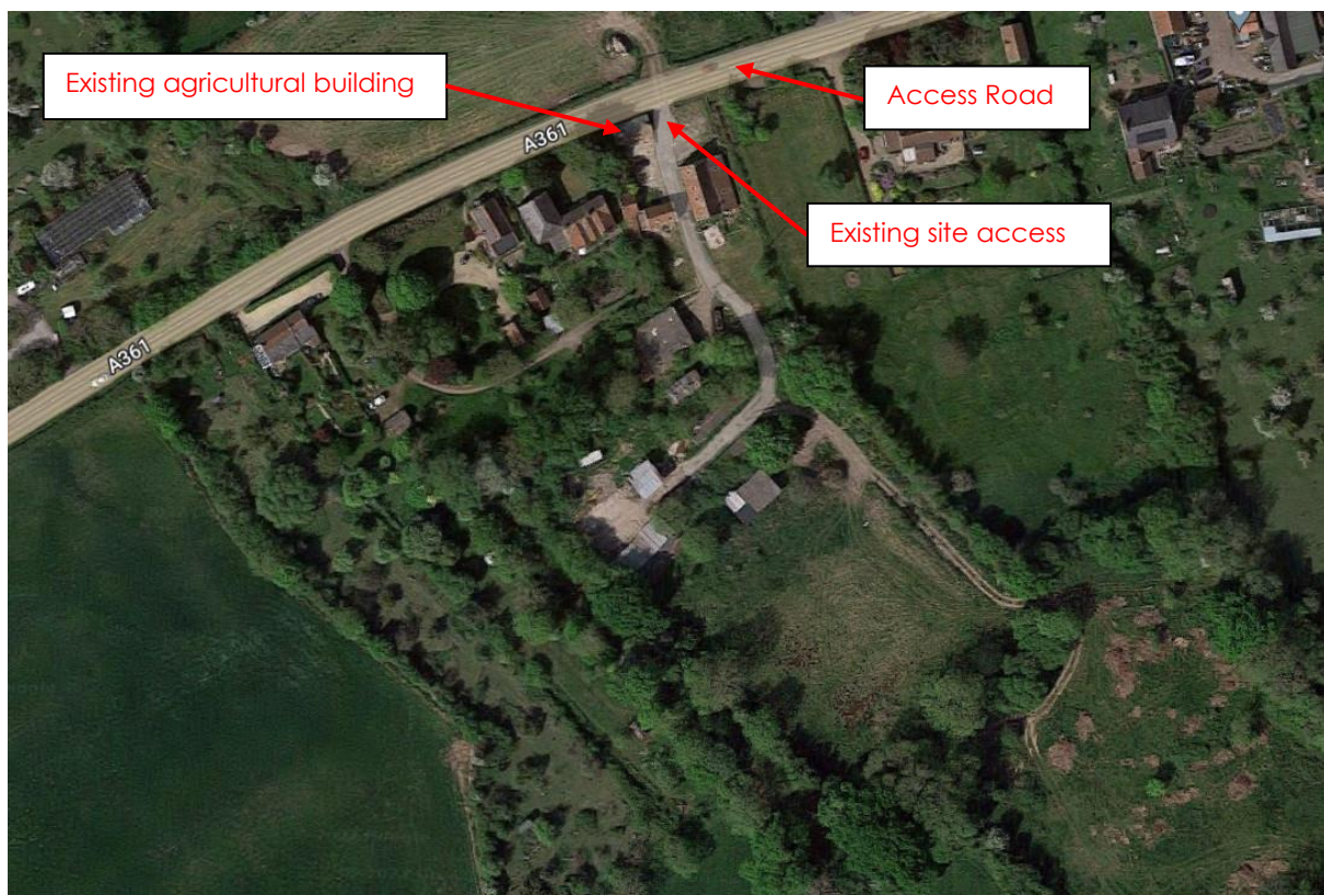
Image 1: aerial view of the existing site and surrounding area
