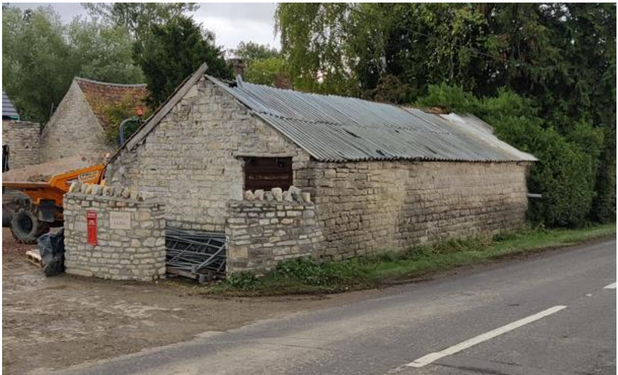
Image 4: North elevation of barn viewed from road.
