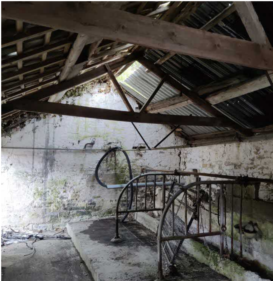
Figure 3 – Internal view looking west
