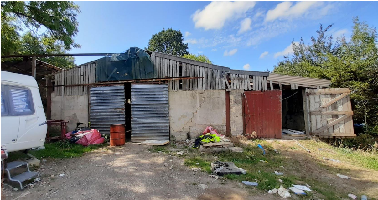
Image 3: East elevation of barn viewed from parking/turning area.
