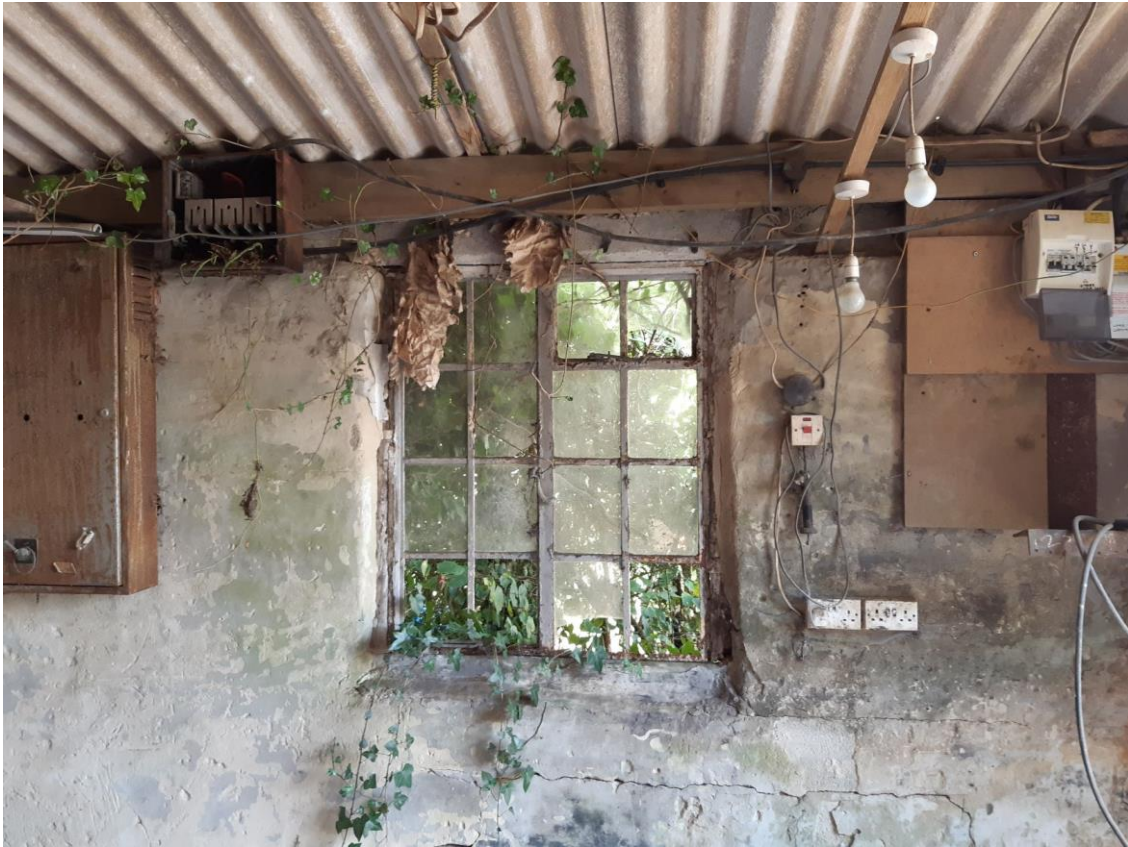
Image 6: Internal view of one of the existing windows to north elevation.
