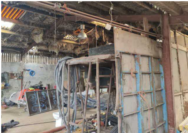
Figure 4 - Internal view of main portal
