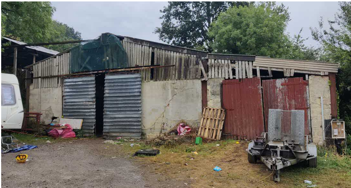
Figure 2 - View from East towards the front of the barn
