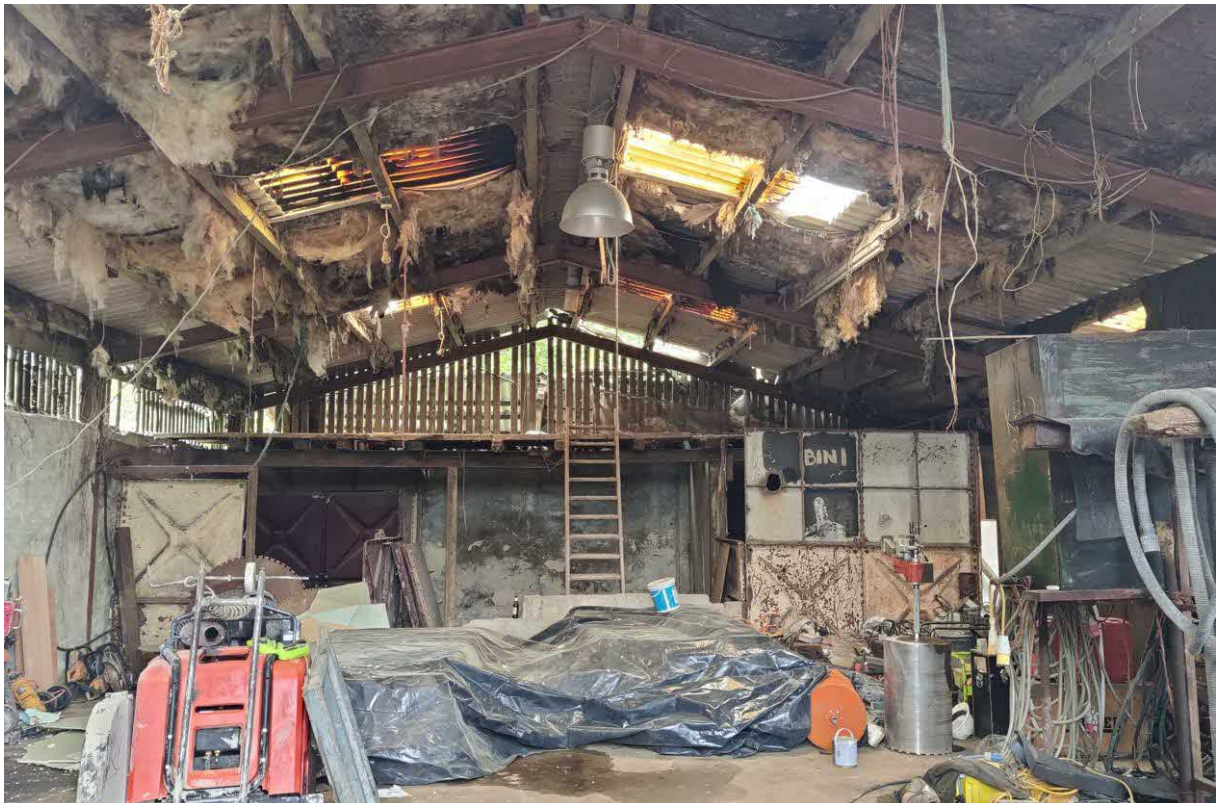
Figure 6 – Internal view from the East
