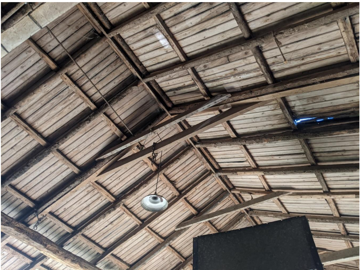
Figure 7 Photo of barn roof
