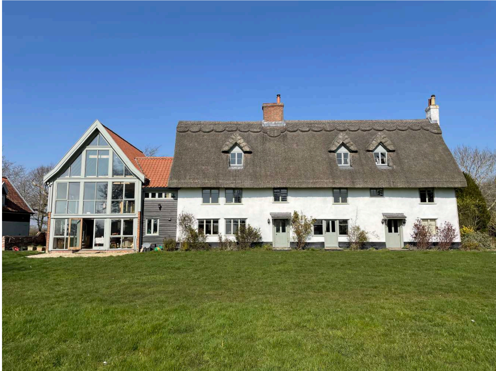
Photo: Showing South Elevation with modern extension and glazed gable.
