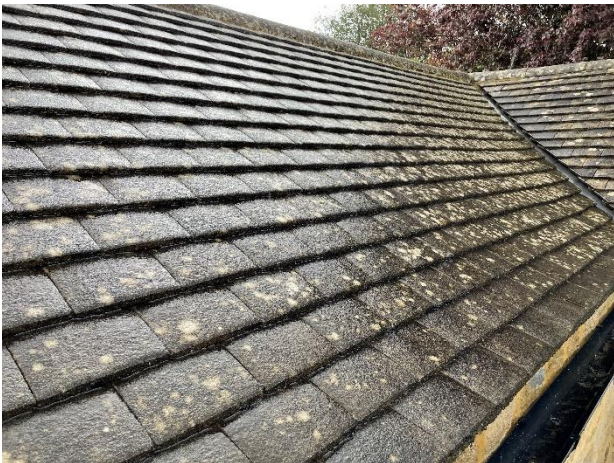
Photograph 5. Detail of the roof tiles.
