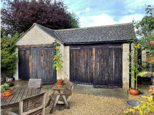
Photograph 1. View of the garage building from the south-east.
