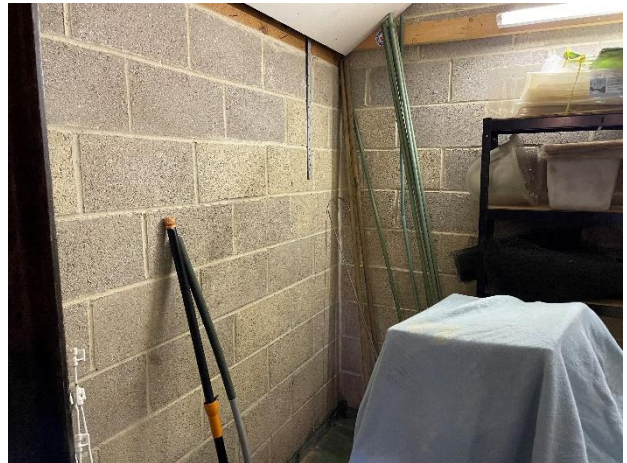
Photograph 4. Detail of the internal concrete blockwork walls.
