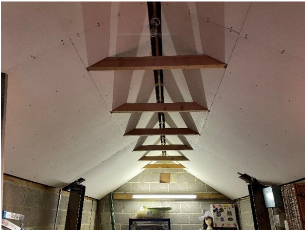
Photograph 3. Detail of the internal roof structure.
