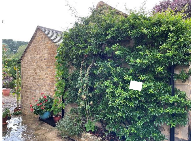
Photograph 2. The two pitched roof sections to the northern side of the building.
