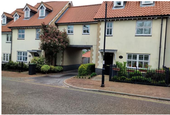
Photograph 7: Recent Co-op site redevelopment shared drive to parking court
