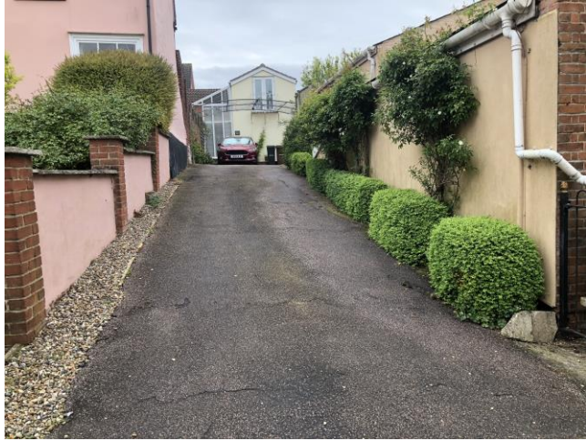
Photograph 6: Shared drive between Pavilion House/ Pump House
