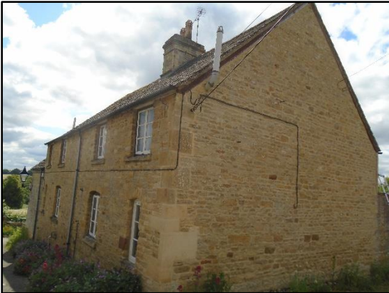
Plate 3: a typical view of the cottage. Photograph showing north-western elevation.
