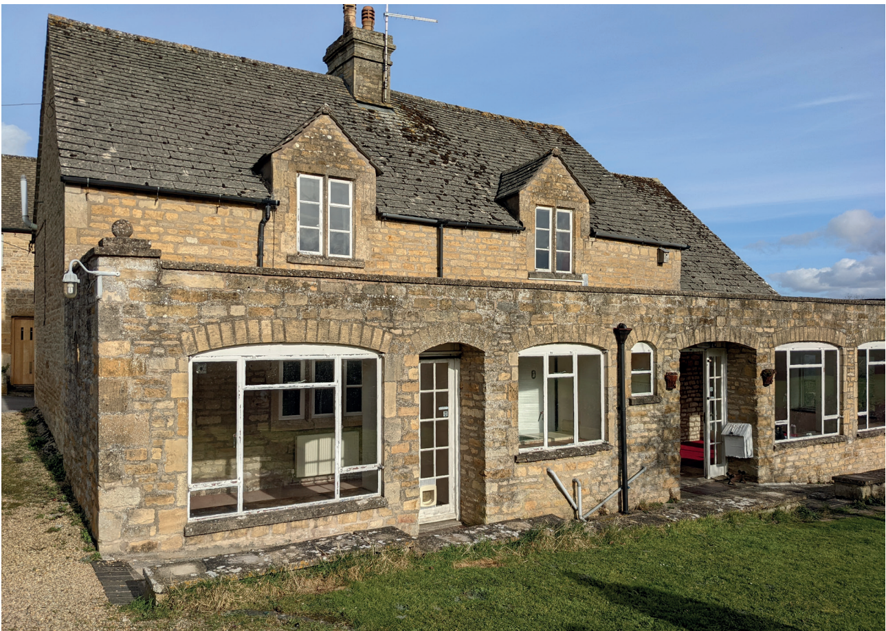
Figure 01 View of existing south elevation with single-storey flat roofed extension
