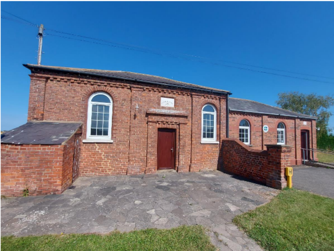
Figure 2- Photograph of existing chapel taken from Lowgate Road
