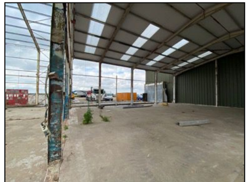
Figure 9 – Internal view of Building 2 looking north-west
