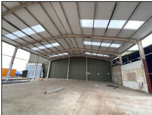
Figure 8 – Internal view of Building 2 looking north-east
