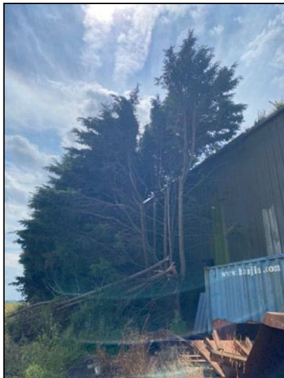
Figure 16 – North-east elevation of Building 5
