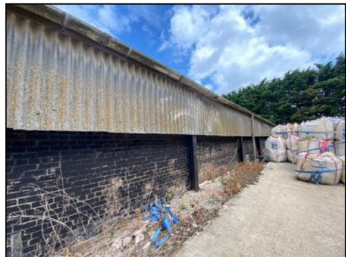
Figure 12 – External view of the south-east elevation of Building 4
