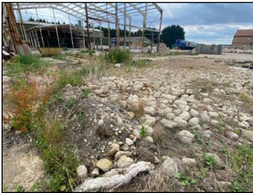
Figure 18 – Area of rubble to the south-west of Building 1
