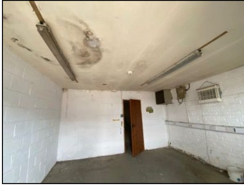
Figure 15 – Internal view of south-west section of Building 4 looking south-east
