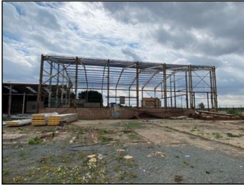
Figure 6 – External view of Building 1 to the north-west
