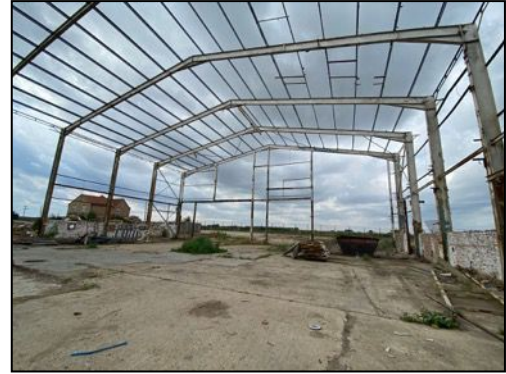
Figure 7 – Internal view of Building 1 looking south-west
