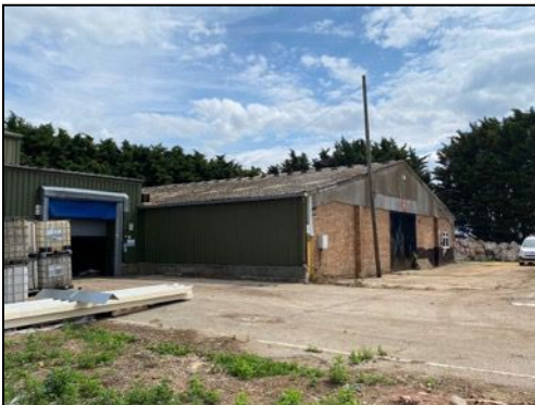
Figure 11 – External view of the west elevation of Building 4
