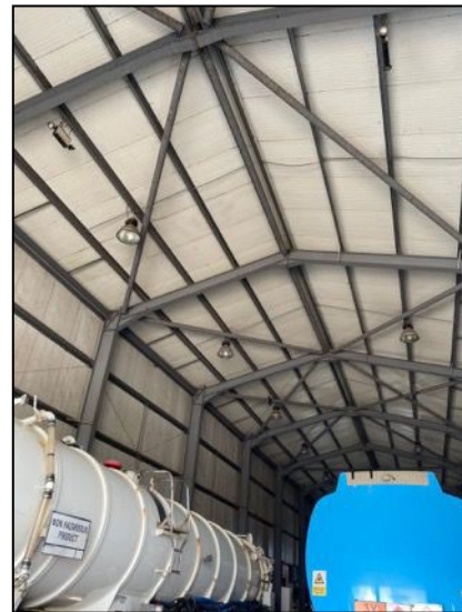
Figure 17 – Internal view Building 5 looking south-east
