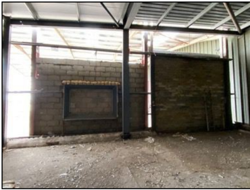
Figure 10 – Internal view of Building 3 looking north-west
