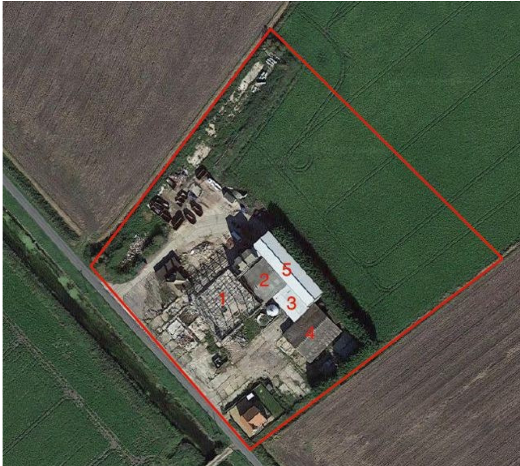
Figure 3: Existing Buildings on the Development Site
