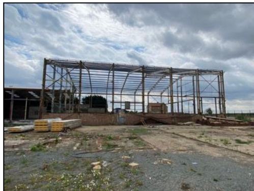
Figure 4 – External view of Building 1 to the north-west
