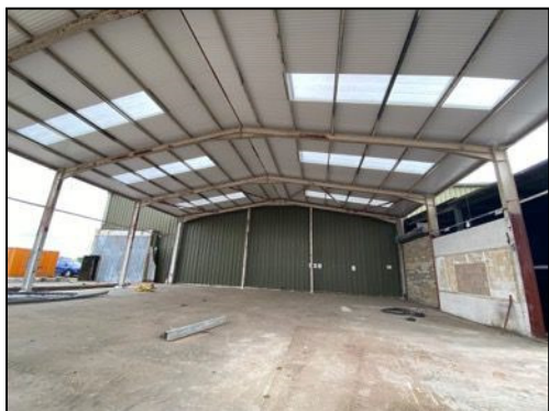
Figure 5 – Internal view of Building 2 looking north-east
