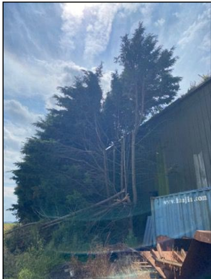
Figure 8 – North-east elevation of Building 5
