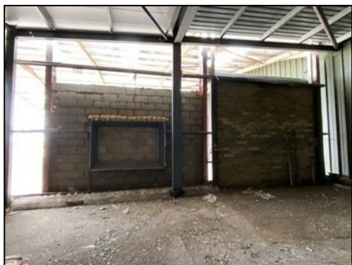
Figure 6 – Internal view of Building 3 looking north-west
