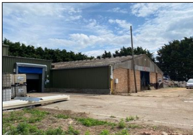
Figure 7 – External view of the west elevation of Building 4
