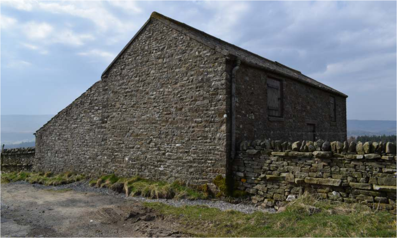
Plate 3. View of the building from the road (looking southwest)
