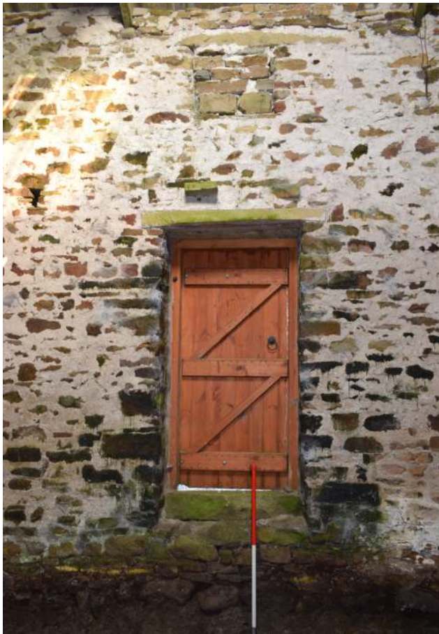
Plate 23. Door D2, internal view with blocked window W6
