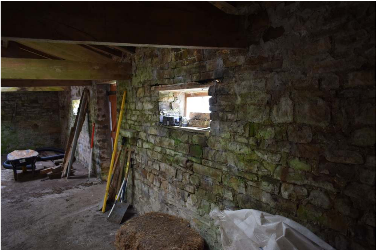
Plate 31 (above). The byre looking southeast
