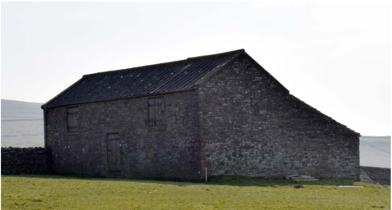
Plate 6. View of the building, looking southeast
