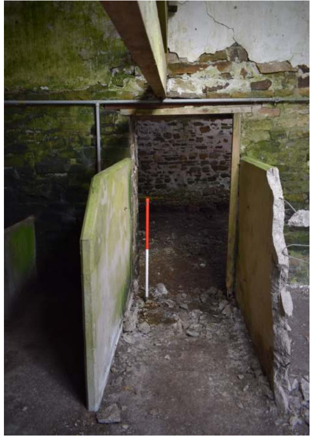
Plate 34. Door D3, view from the byre
