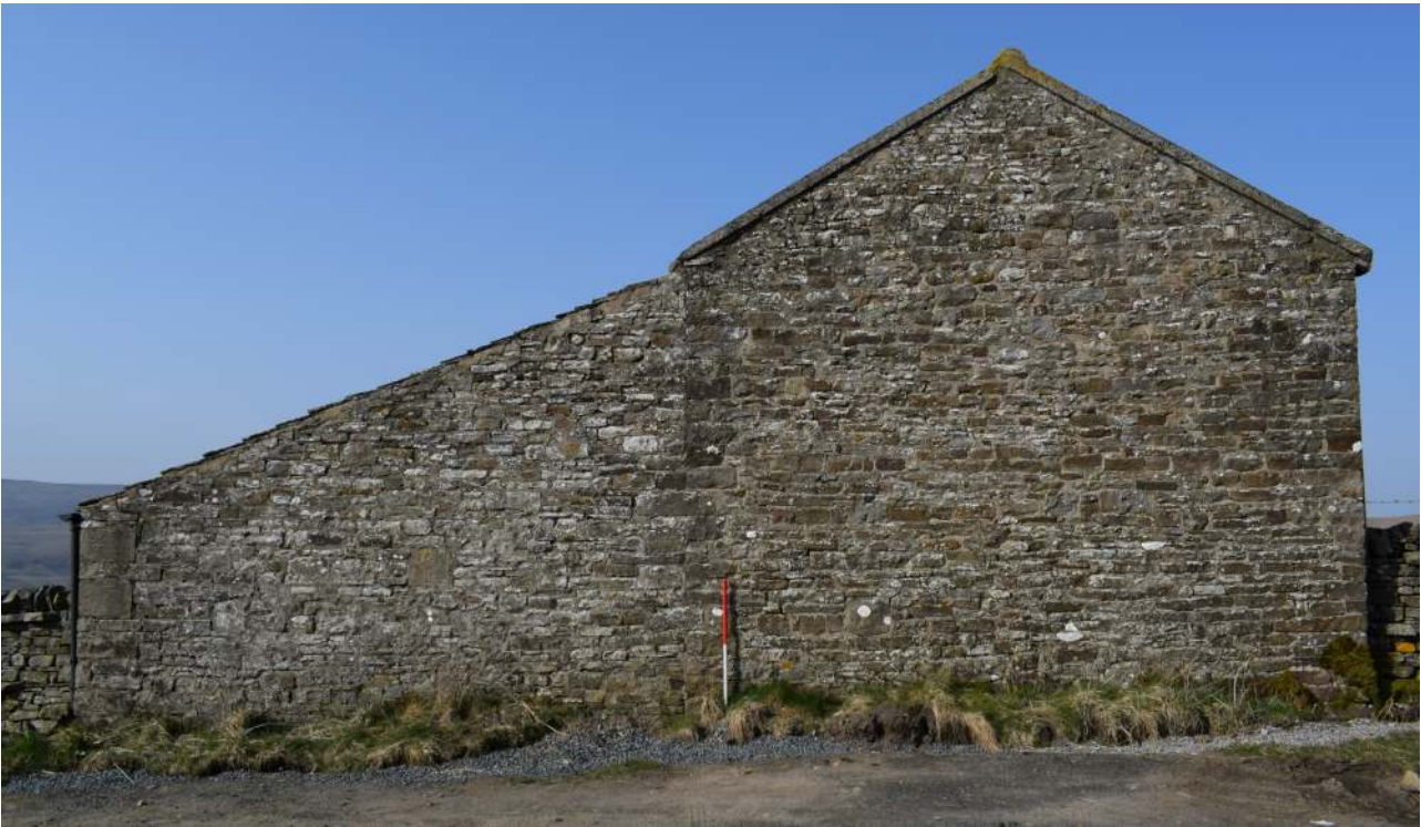
Plate 7. The east-facing elevation as seen from the road
