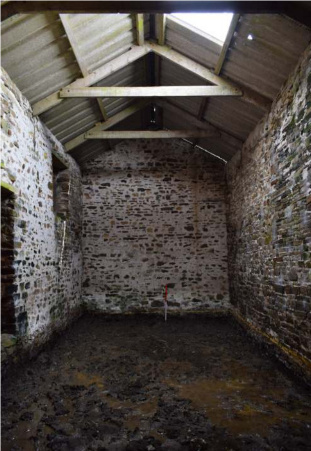
Plate 19. Northern room, looking east
