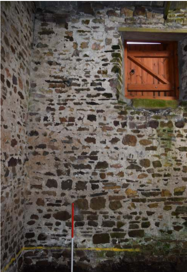
Plate 25. Window W5 internal view
