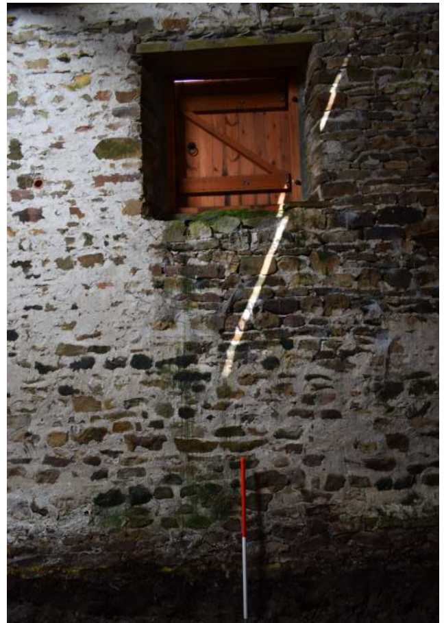
Plate 24. Window W4, internal view
