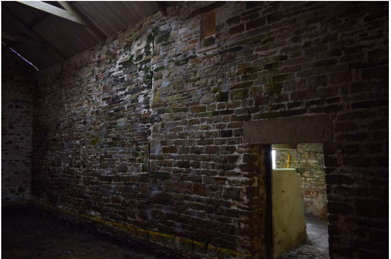
Plate 22. Northern room, looking southeast
