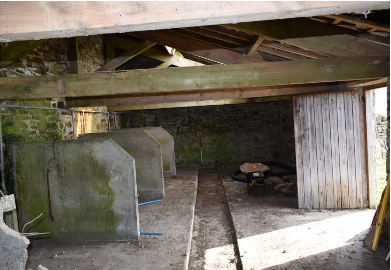
Plate 29. The byre looking east
