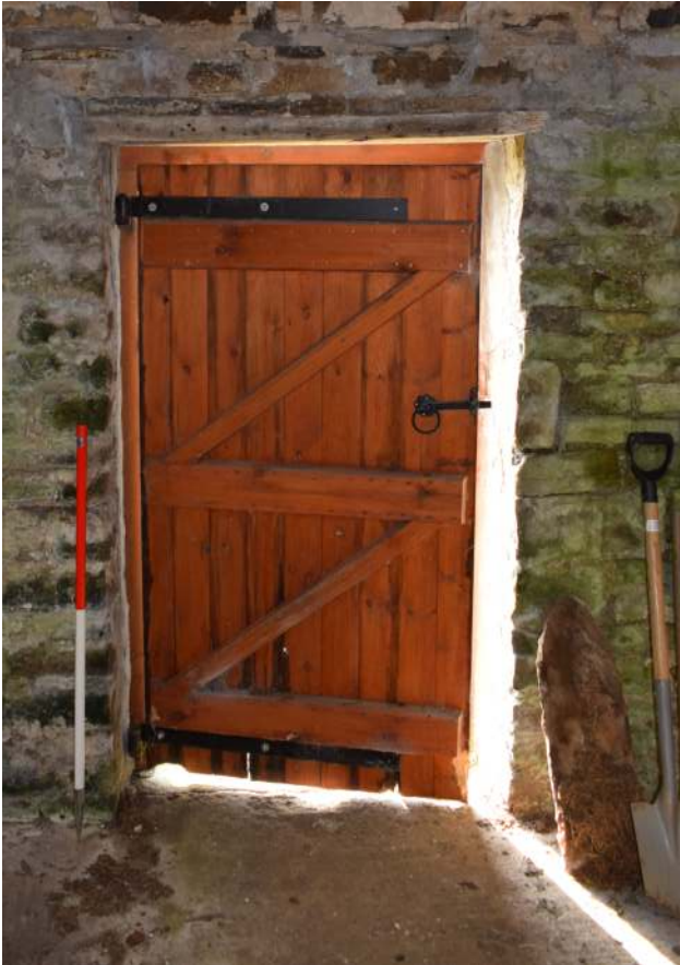
Plate 39. Doorway D1, interior
