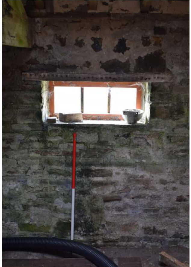
Plate 40. Window W1, interior
