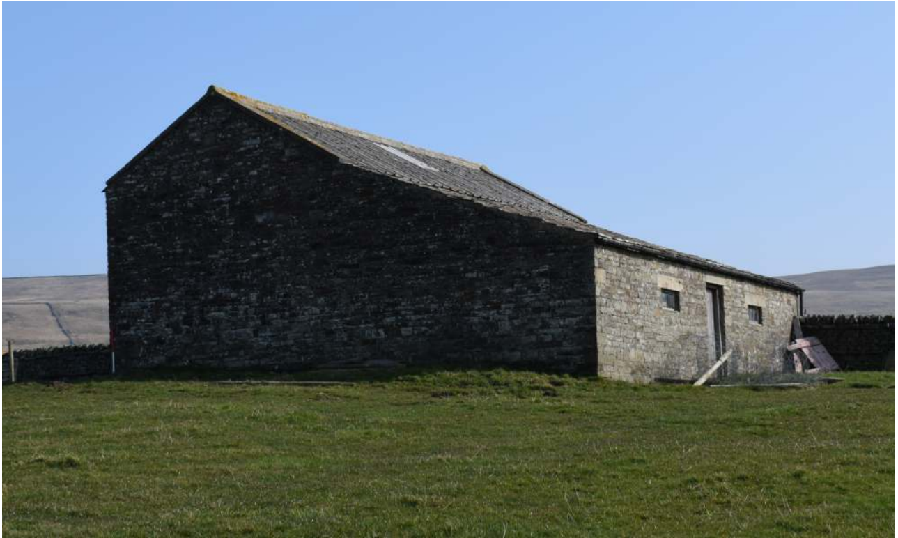
Plate 5. View of the building, looking northeast
