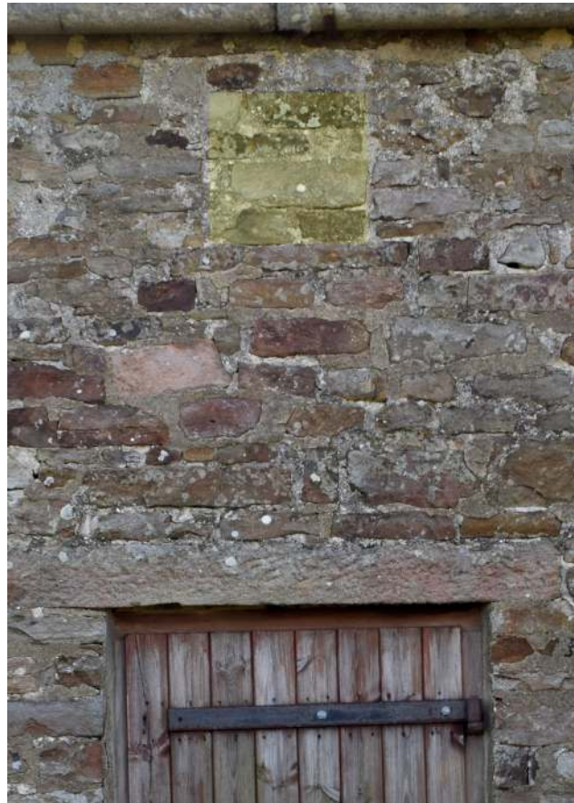
Plate 18. Northern elevation, blocked window, W6
