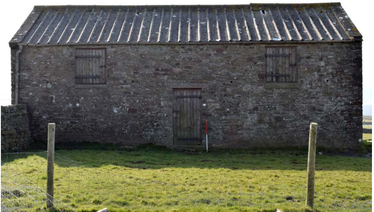
Plate 14. The north-facing elevation
