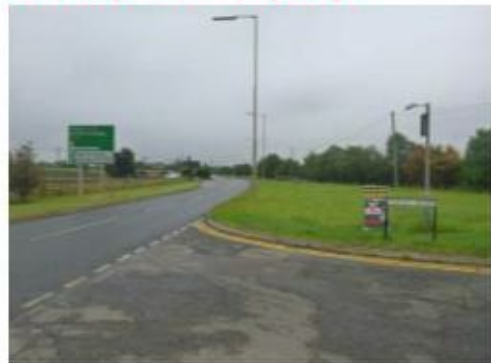
Photo 3.4 Old Tilbury Road visibility to right
