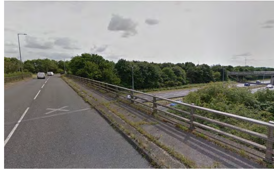
Figure 5 – View from A128 approach
