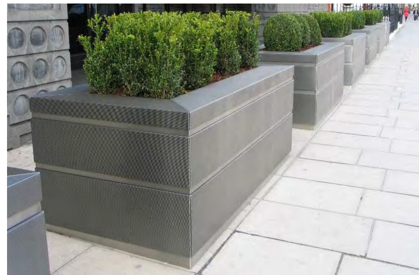
Example of planters that are used for securing building perimeter at ground level
