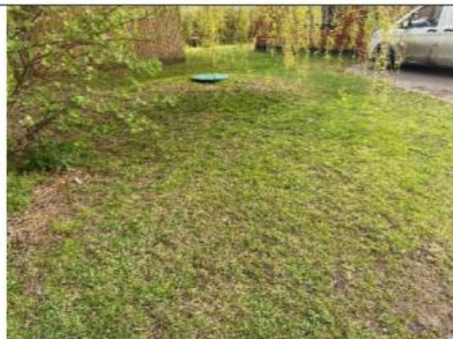
Photograph 13 Below ground LPG tank in residential garden.
