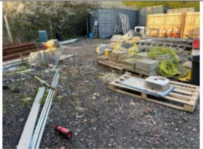
Photograph 02 Shipping containers / materials storage NE corner.
