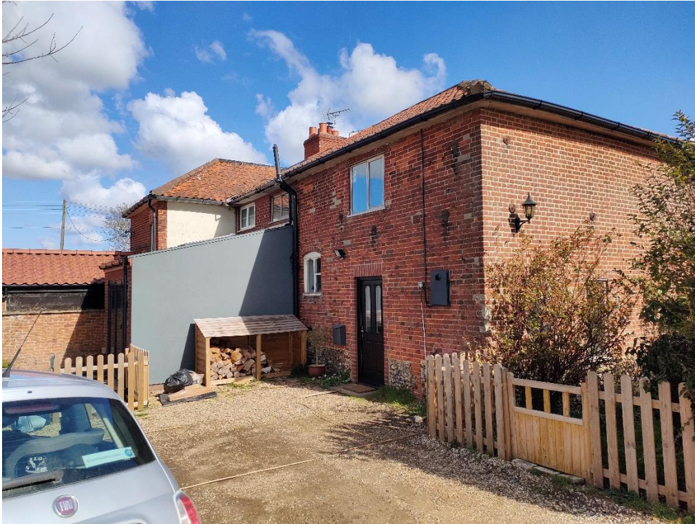
View from access track onto main Dwelling
