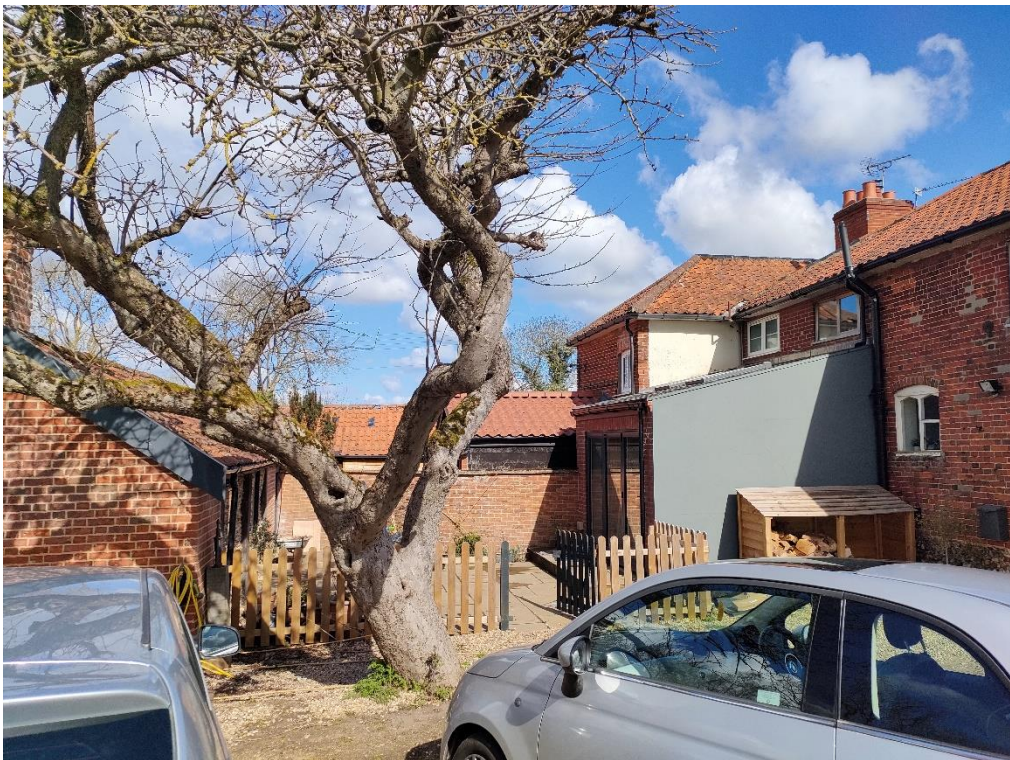
View from access track onto side of outbuilding and dwelling. Please note position of tree to be removed.
