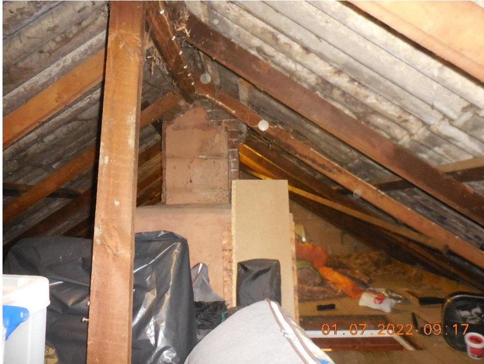
Photo 2: Interior of roof space in cottage.
