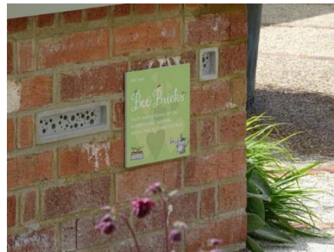
Bee Brick - case in concrete: 215mm x 105mm x 65mm
