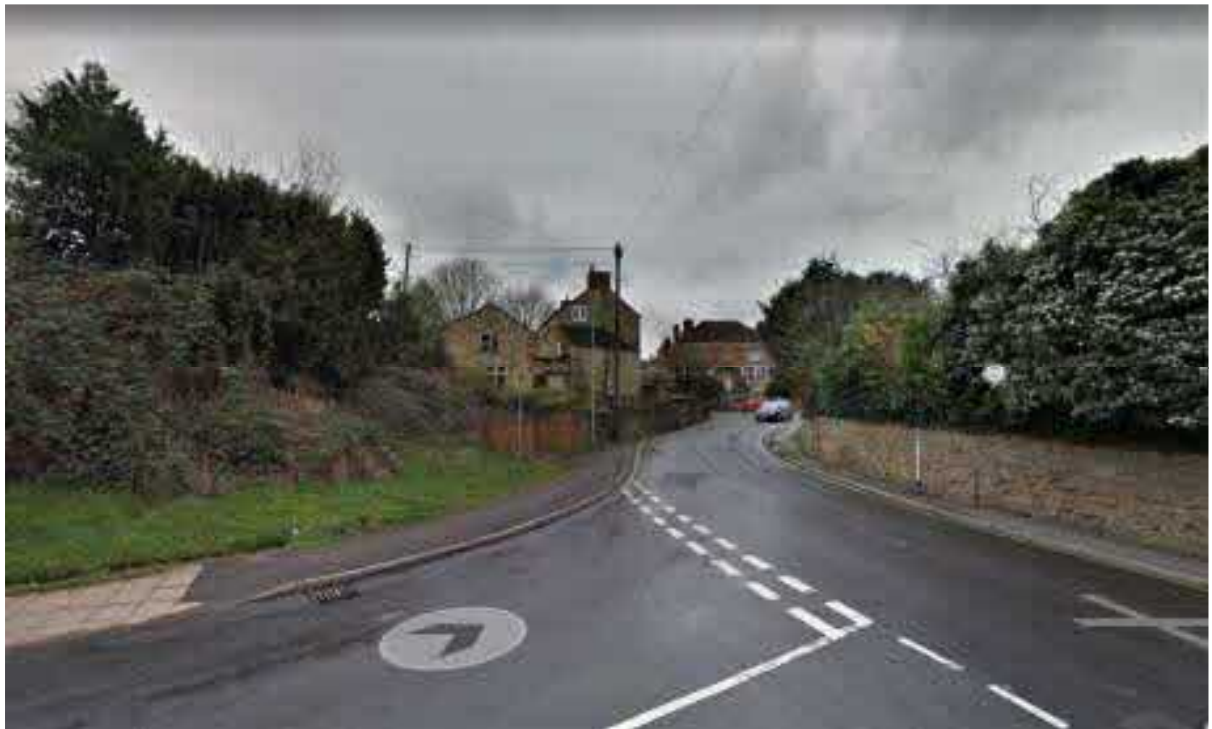
Fig 6: Principal view of the house from Station Road. Note the elevation of the building to the immediate right of Red House Farm.
