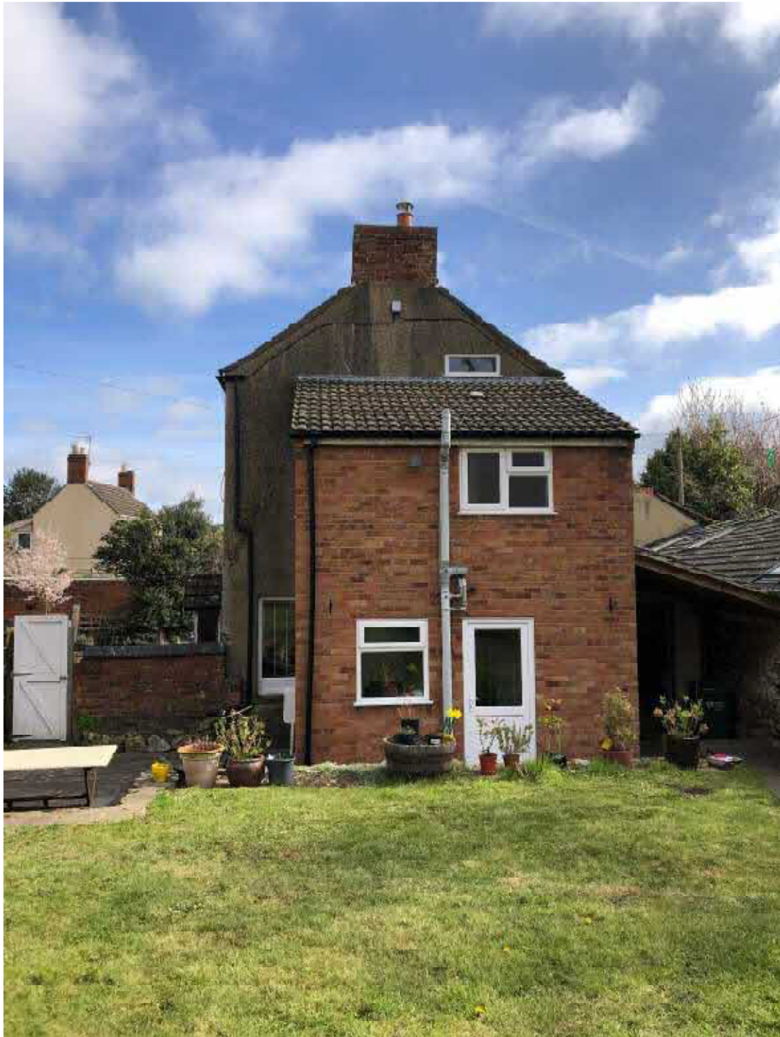
Fig 5: View from rear garden towards the south-west gable and modern extension. The roof over the covered area at the rear of the house can be seen on the right.
