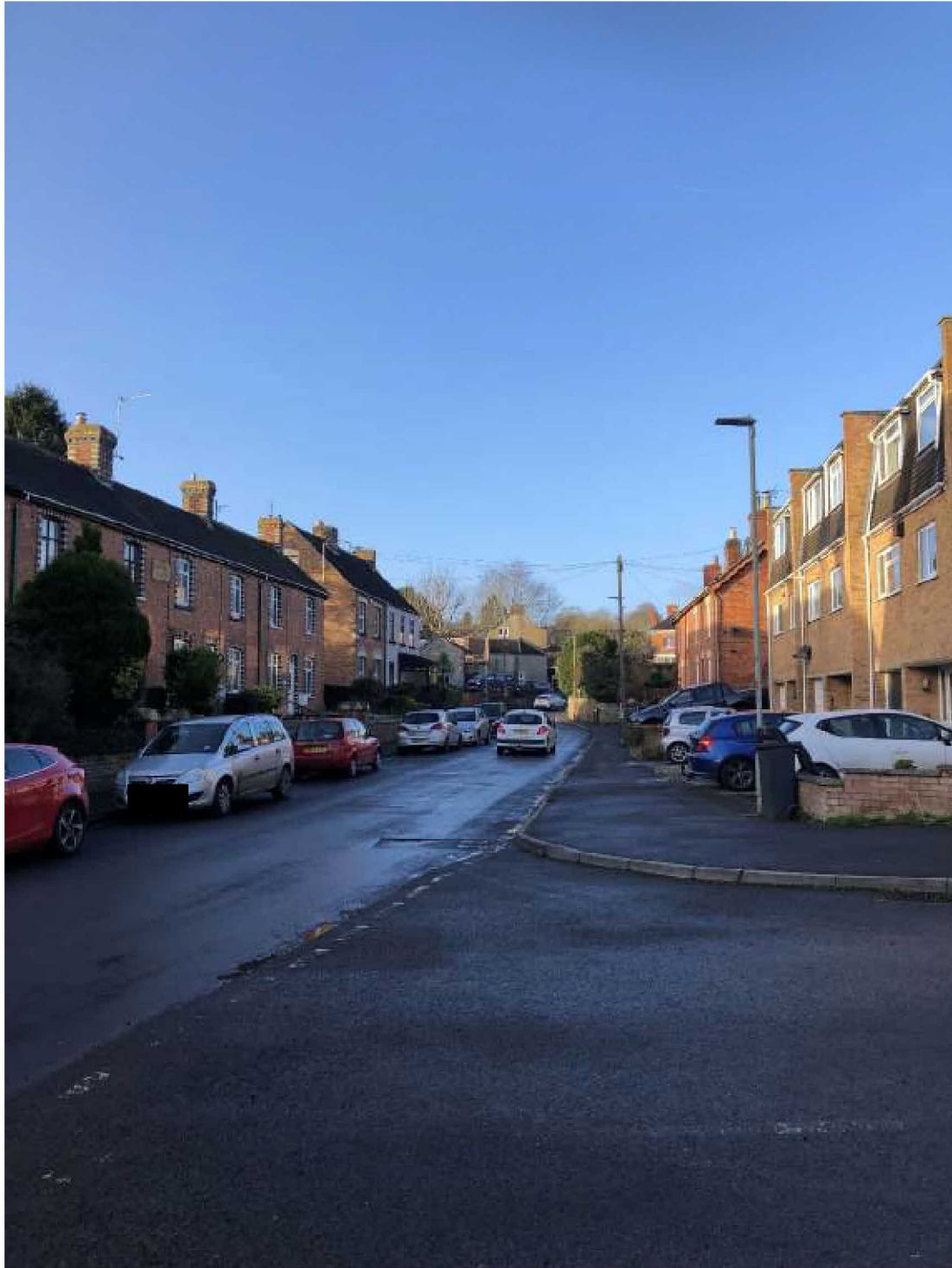
Fig 12: View from the Railway pub on Station Road putting Red House Farm in context.
