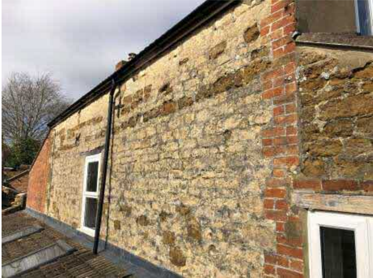
Fig 1: Rear elevation of the main house showing natural stone wall and brick quoins and the existing roof over the rear of the house.
