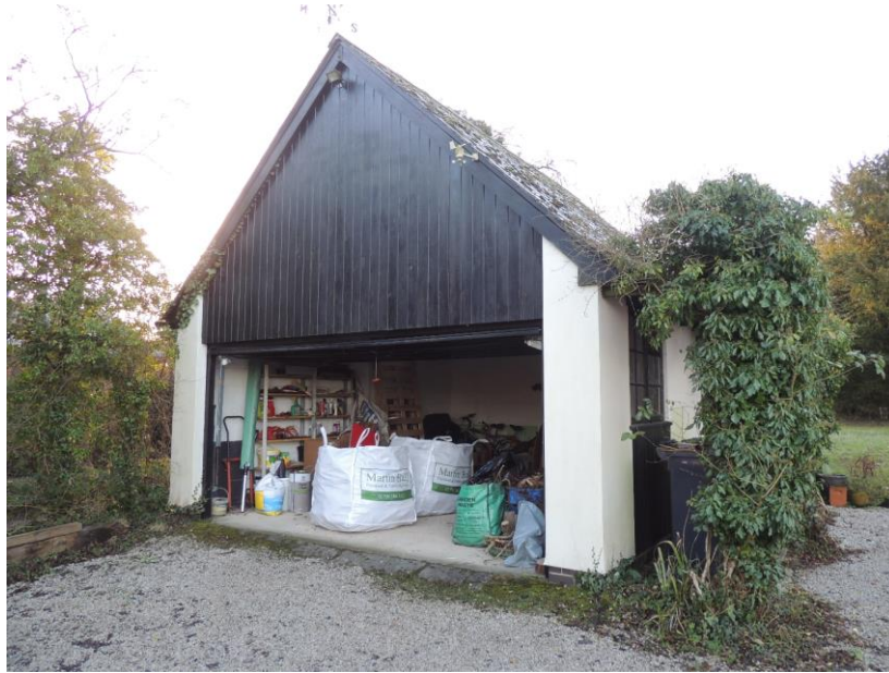
Photo 1: Northern elevation. The proposal is to demolish and replace the garage
