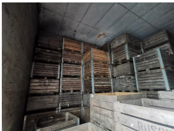
Interior areas of cold store
