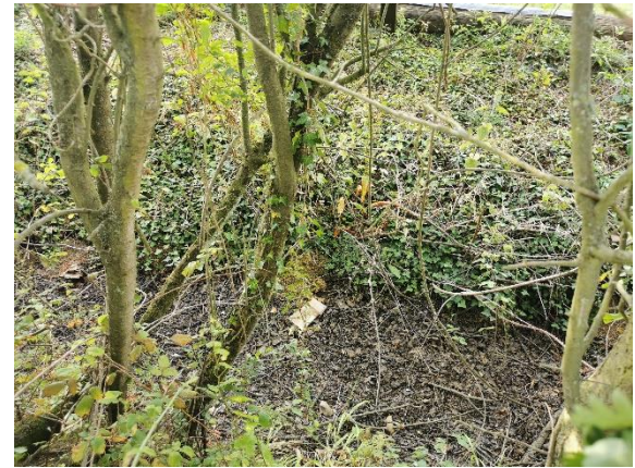
Dry ditch that was heavily shaded
