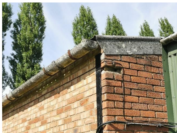
Lifted panel at the top of the roof
