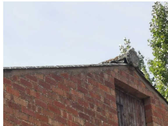
Lifted panels at the ridge
