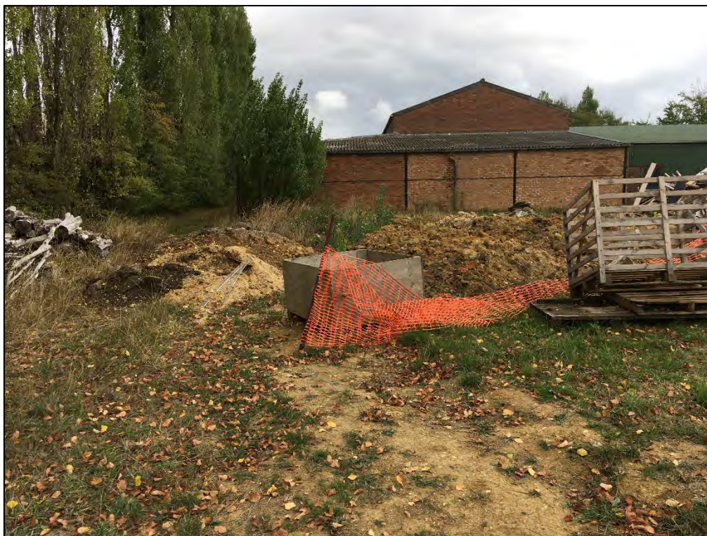
Photograph 16: Piles of logs, pallets, soil etc. to the rear of the buildings, i.e. within the western sector of the site.
