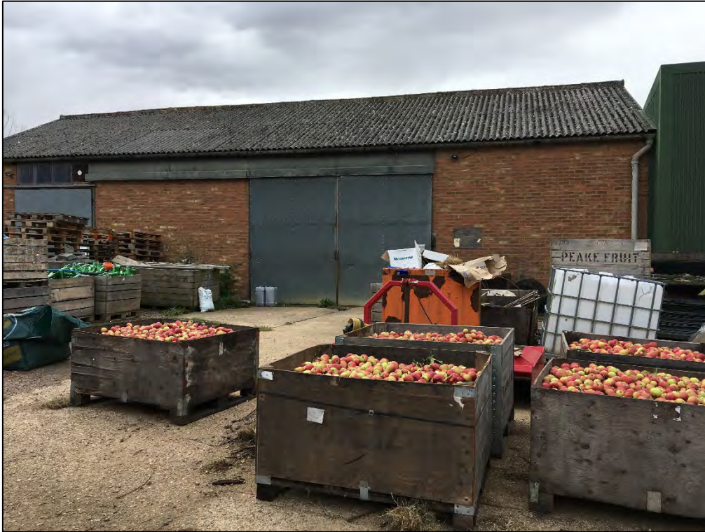
Photograph 11: The workshop building adjoining the buildings on-site.
