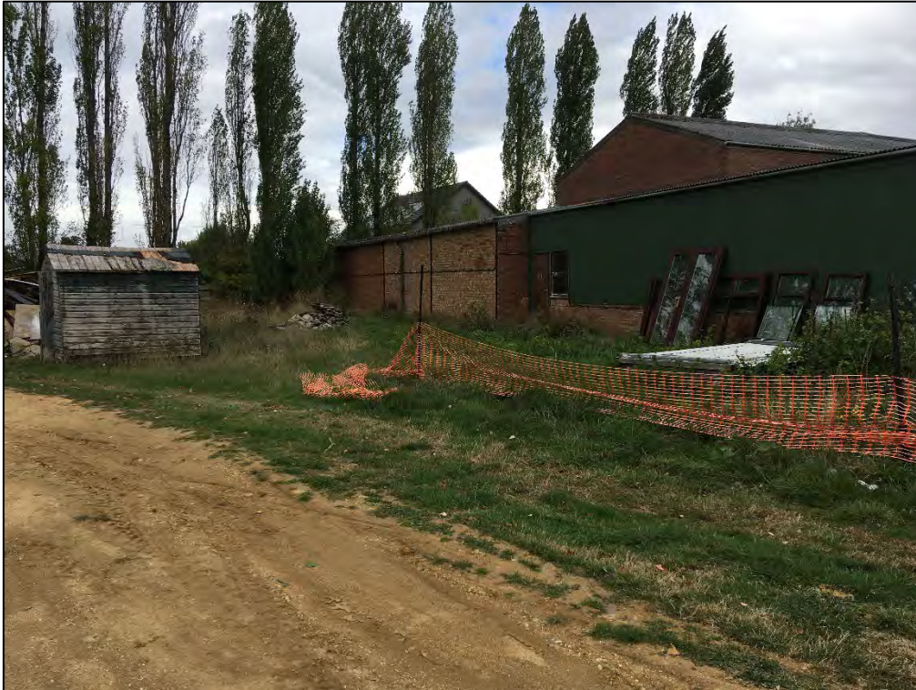
Photograph 15: The area to the rear / west of the buildings, which was covered in grass and in use for the storage of building materials and materials arising from the development of land to the north.
