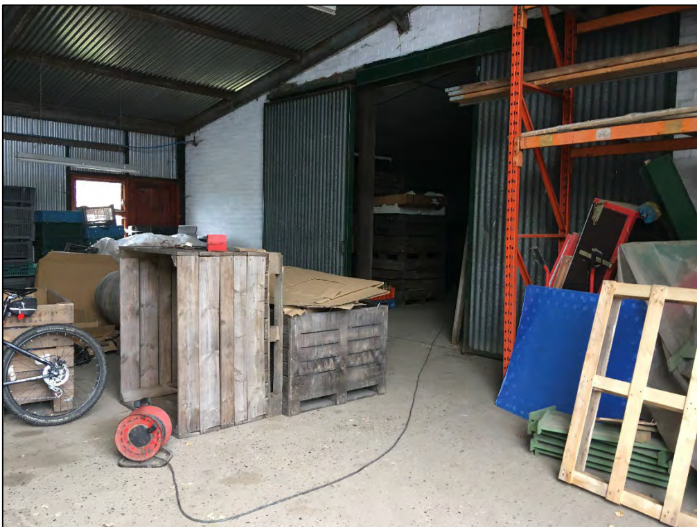
Photograph 10: Inside the green metal sheeting building.
