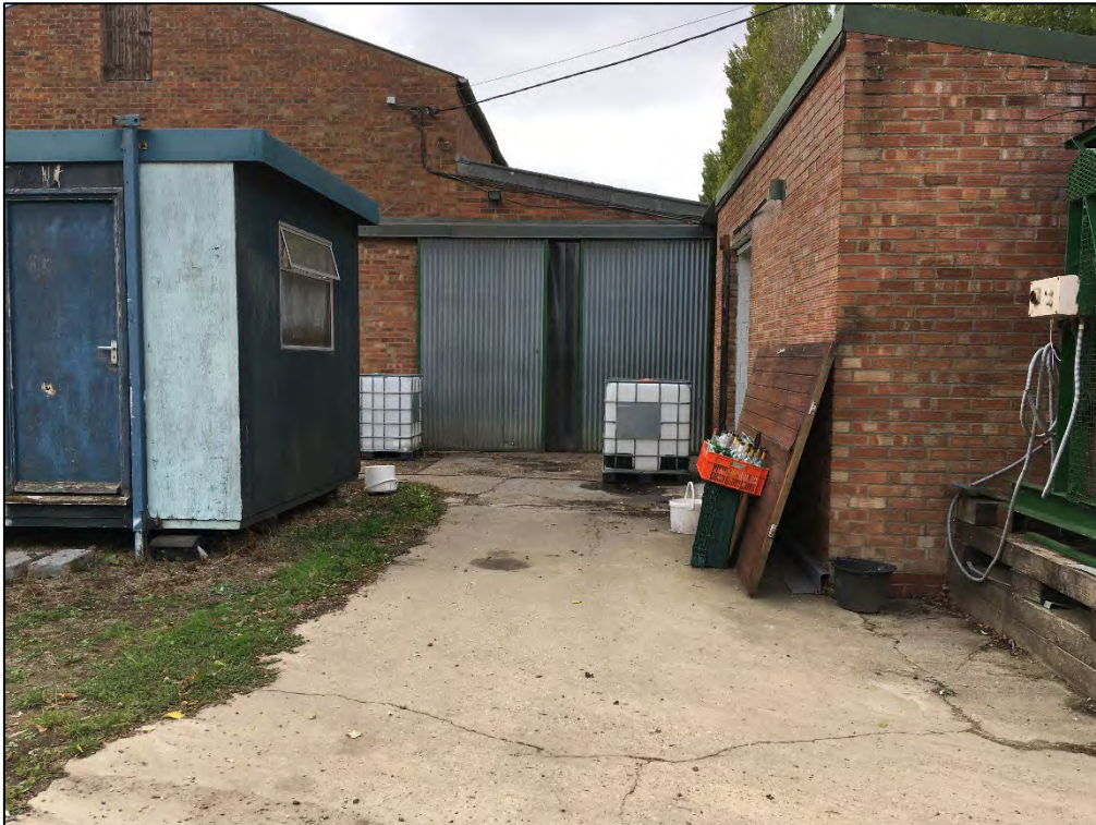
Photograph 4: The adjoining lean-to to north of the large barn, a small brick building in use for pressing apples and a small portable wooden building in the north-east of the site.
