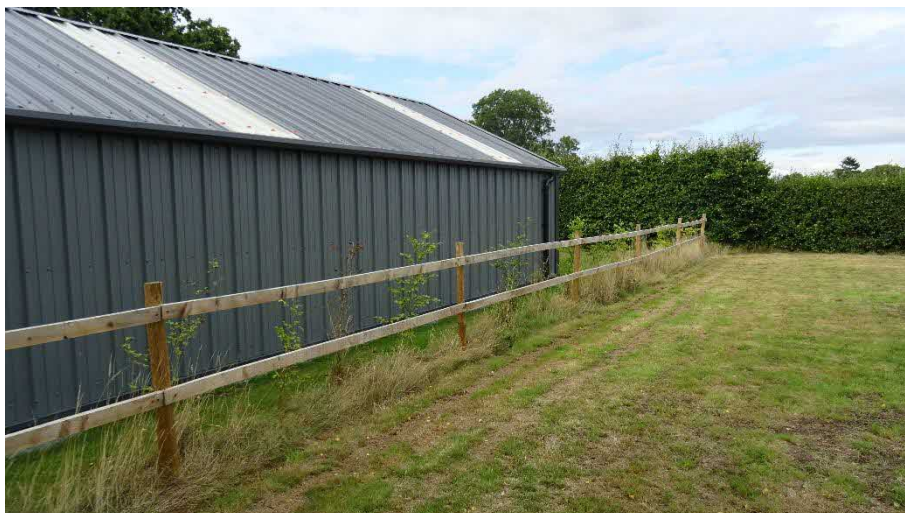
Figure 4.6. Wooden fence to the west
