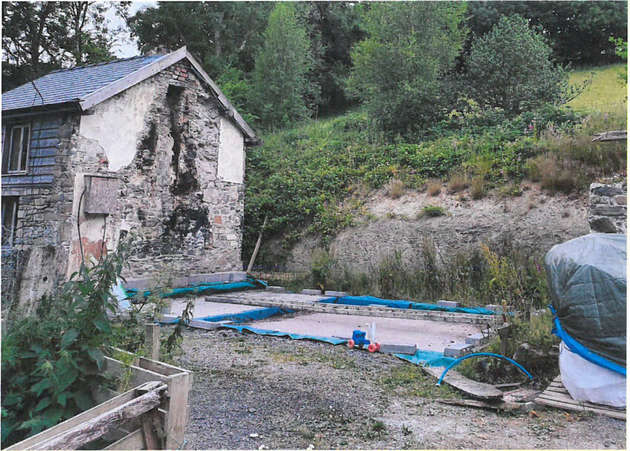
Figure 2: The eastern gable and foundations for new extension at Longhill
