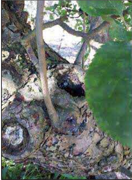
Photograph B4: Apple tree T4 with rot holes leading to an assessment of low bat roost potential.
