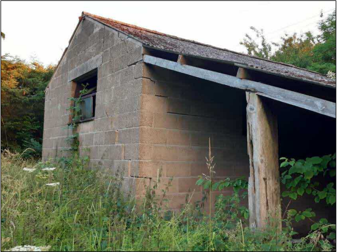
Photograph 6: Northern elevation of the breezeblock storage building (TN1)
