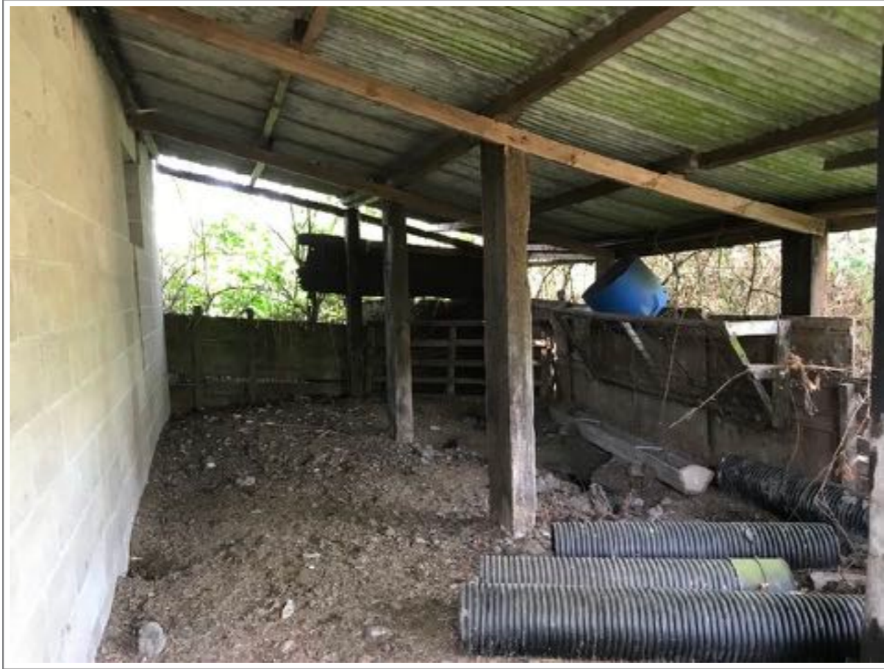
View of open barn looking South East.
