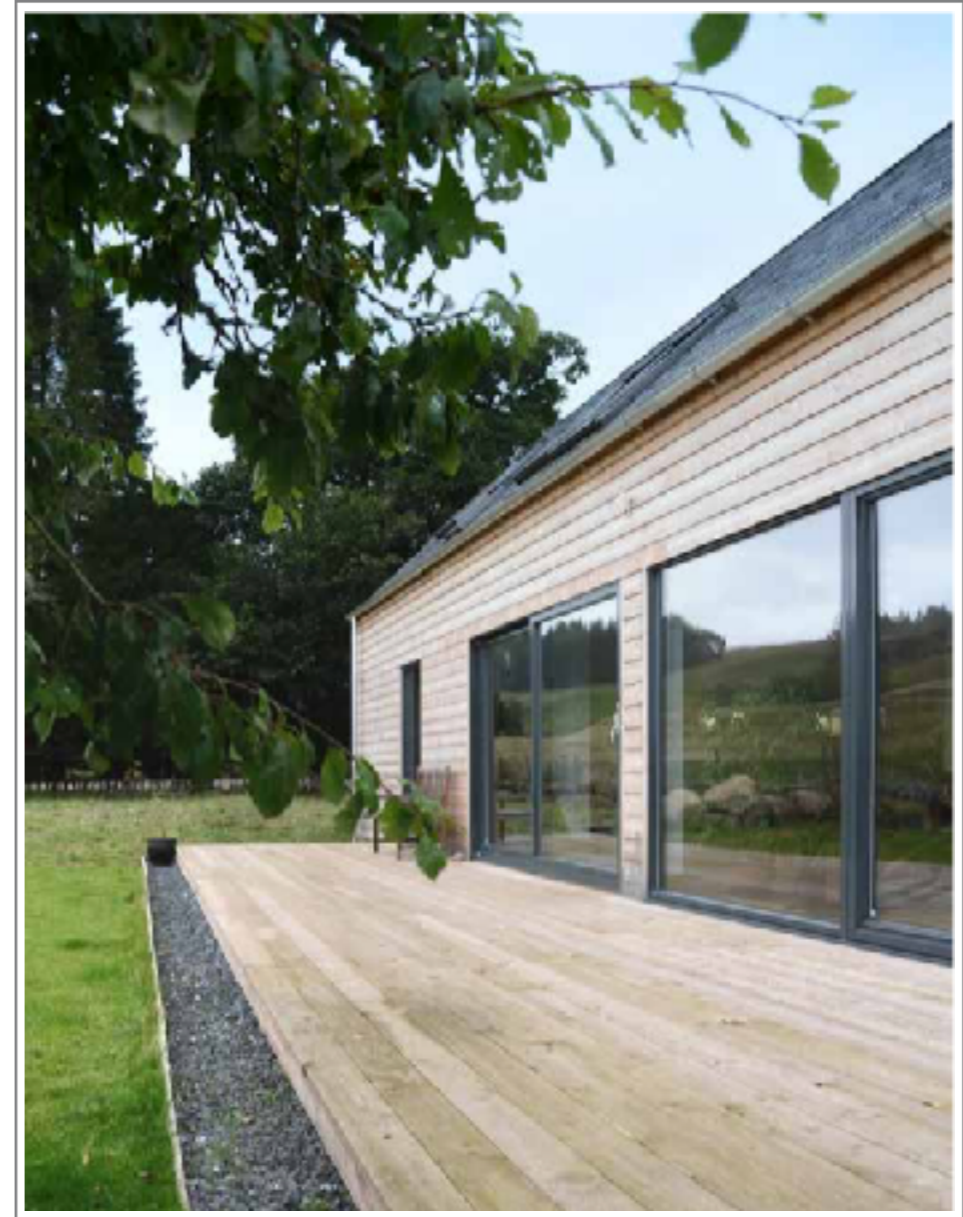
Outside sitting area to be decked in natural timber slightly raised above the ground level.
