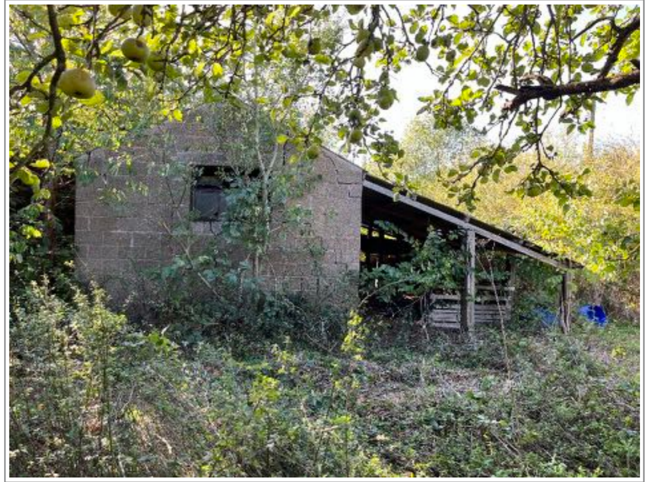
View of existing building North West gable.
