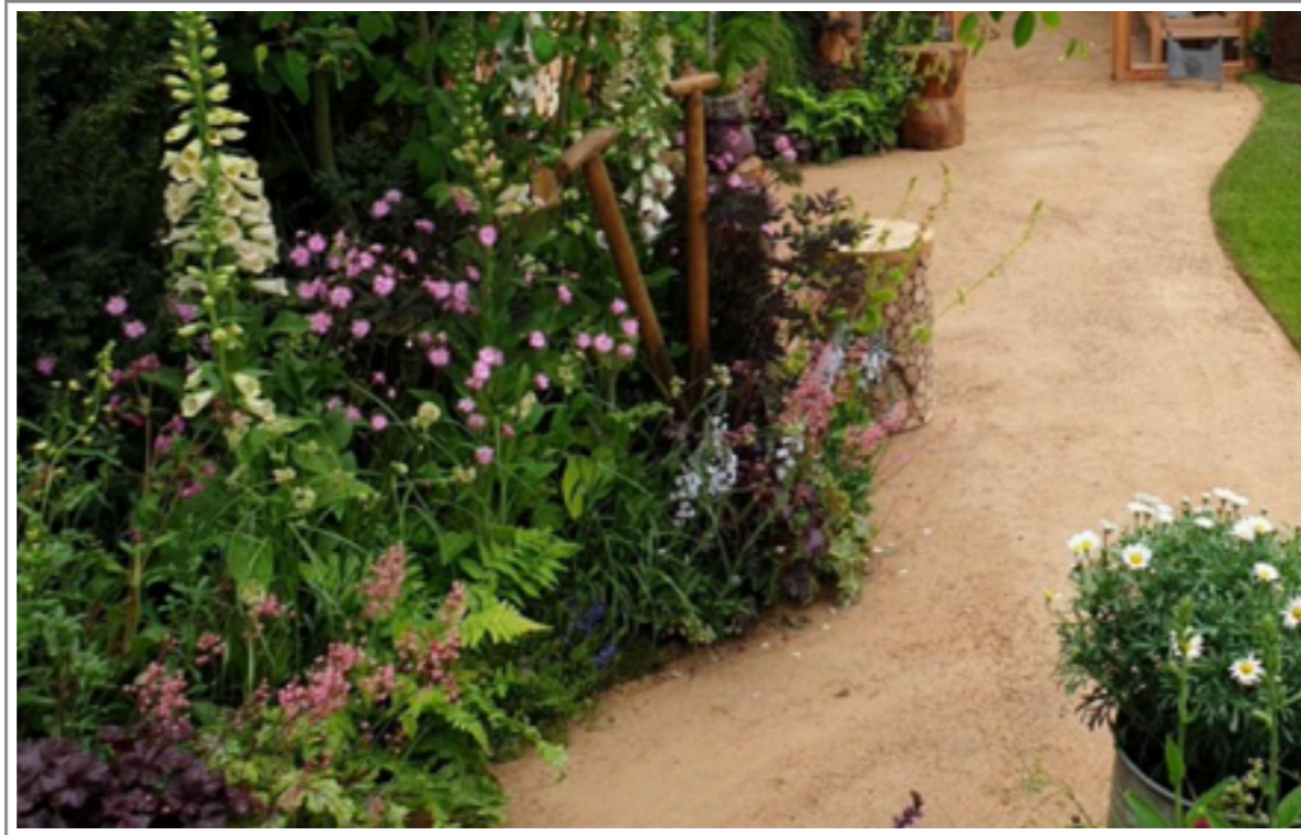
Rolled Breedon gravel parking court and footpaths where shown on drawing no. 307/09.
