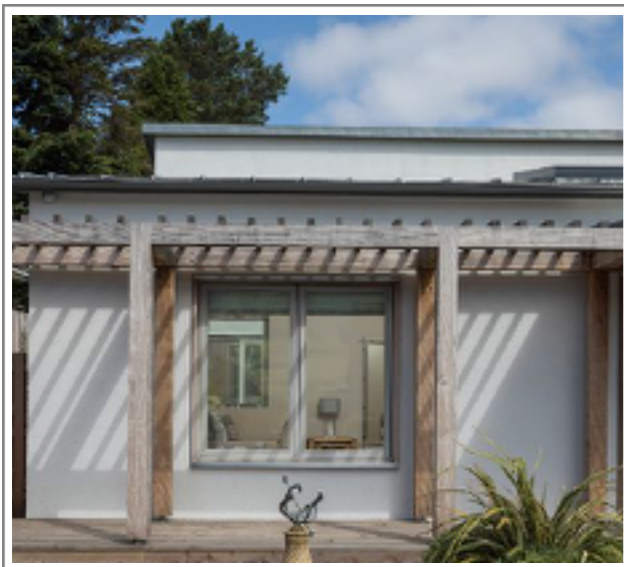
Pergola constructed in a similar manner to thesis pictures formed with substantial sections of timber. Tensile solar reflective fabric can be fitted to sunny aspects.
