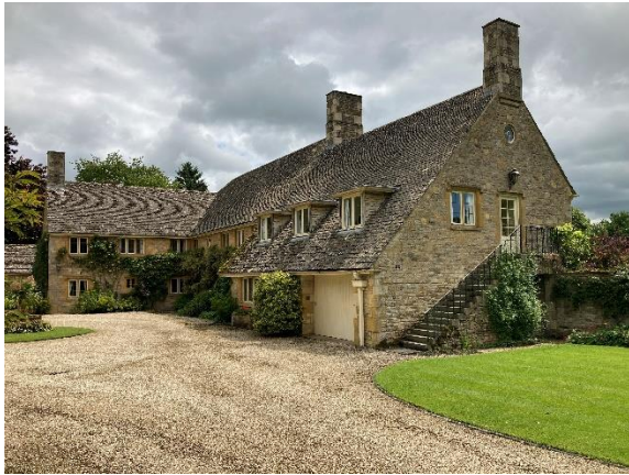
Figure 3 - main house at the site
