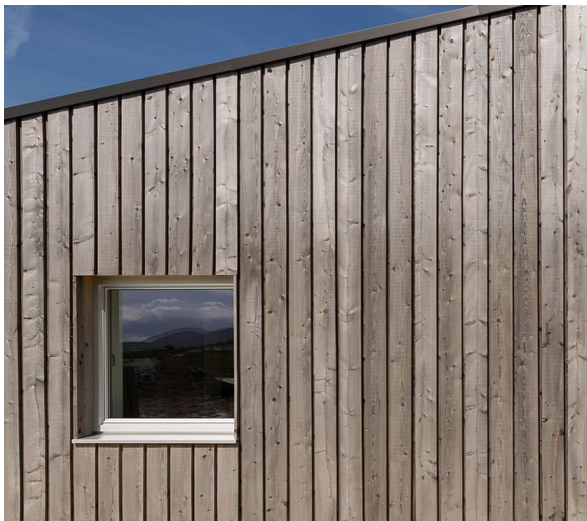
Example of weathered vertical timber cladding
