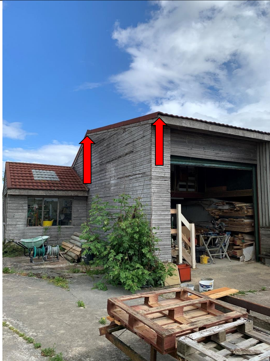
Figure 1: The southwest aspect of the workshop within B1. The red arrows highlight the emergence locations of the two common pipistrelles.
