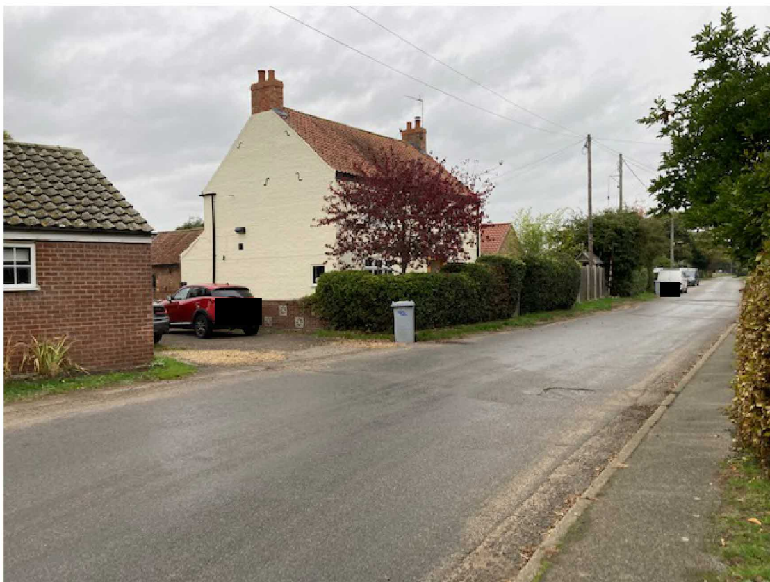
6. Looking north along Thorney Road across the front of Holly Farm.
