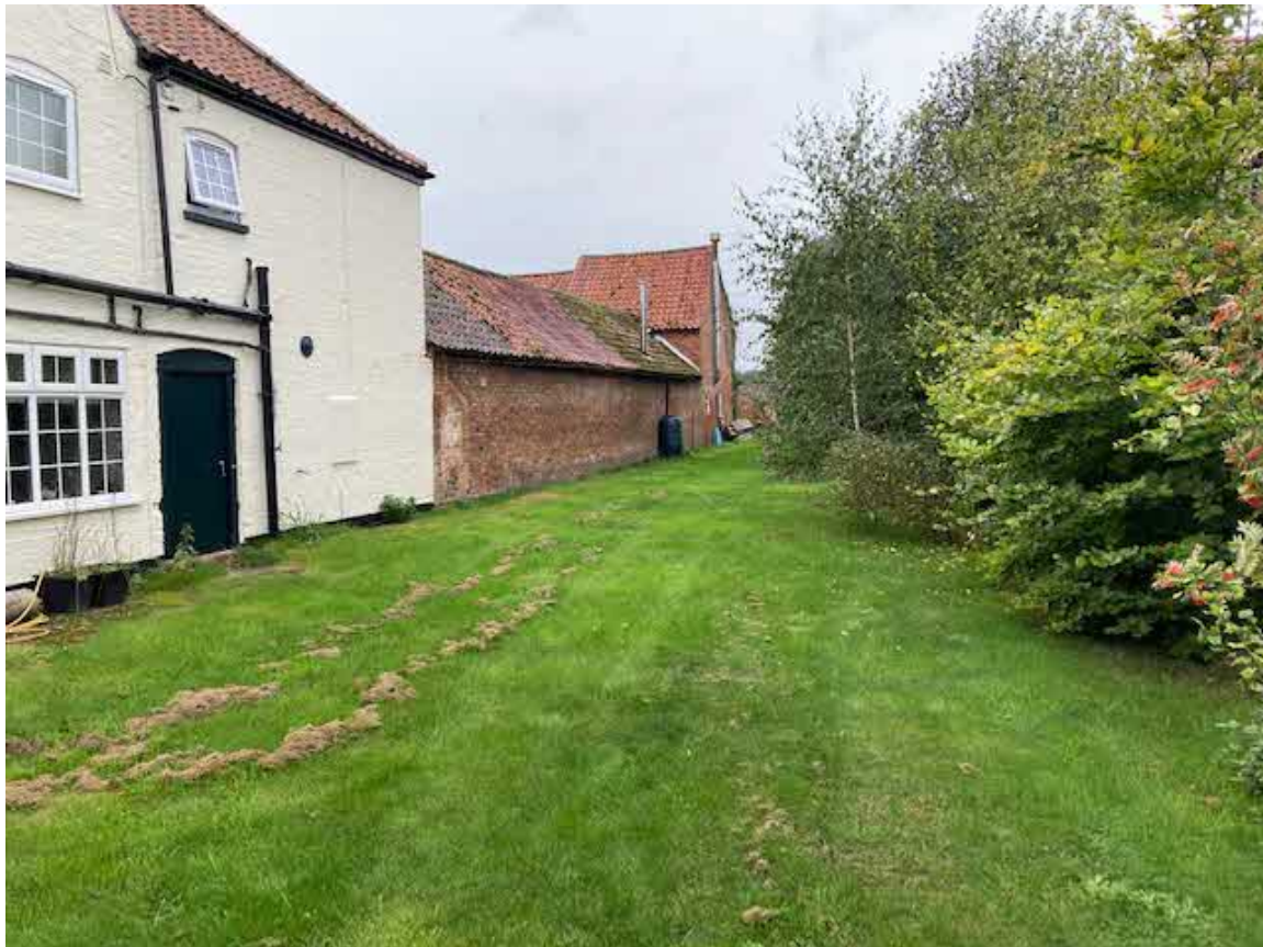
3. Looking west down the north side garden area.
