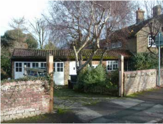
Fig 5. View of front elevation
