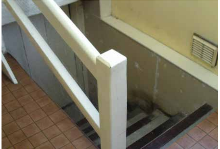
Fig 9. Internal view of basement stair
