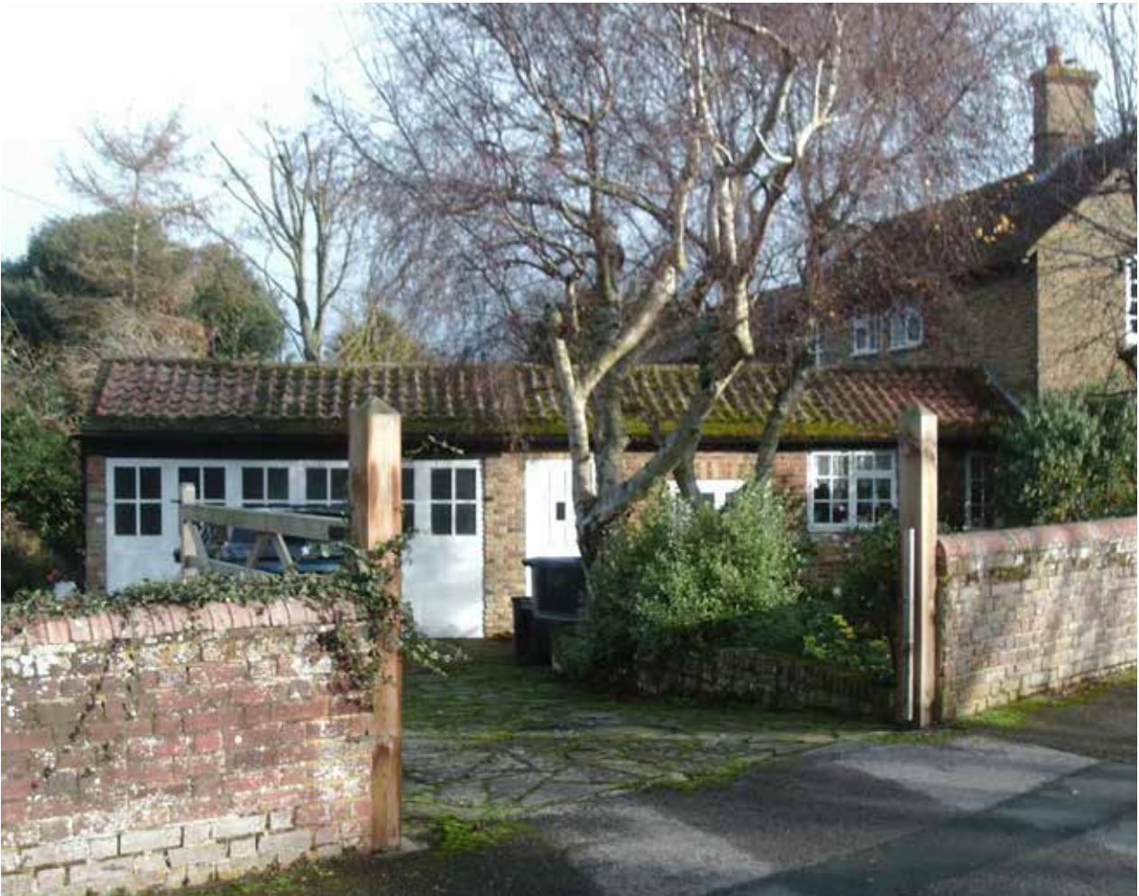
Church Cottages from Court Lane
