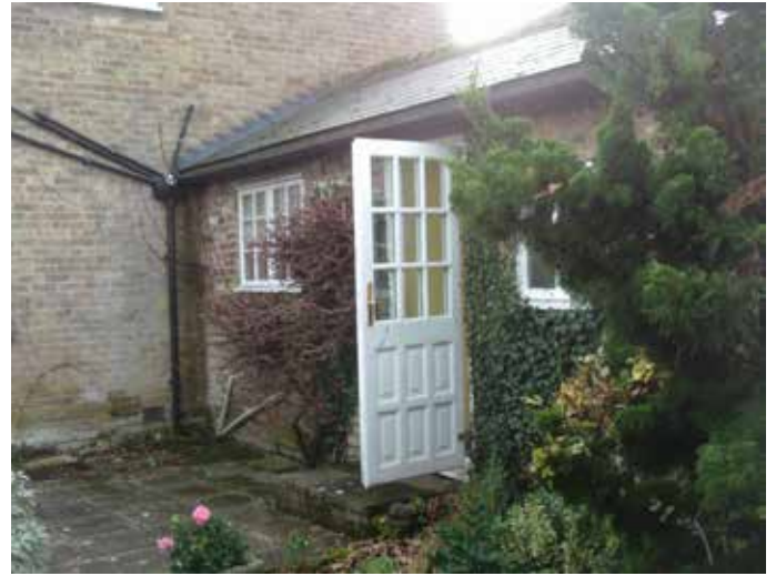
Fig 6. View of rear elevation
