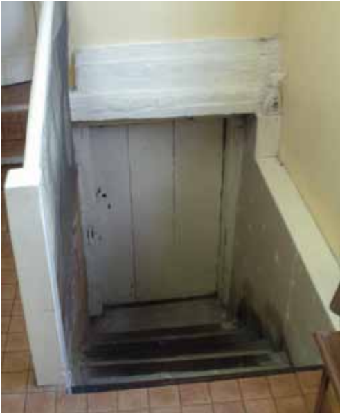
Fig 8. View looking down towards basement entrance
