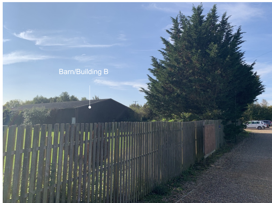
Plate 3: Looking south showing the eastern site boundary between Fairways and the golf club car park and access road. Building B, the Barn to be retained is indicated.
