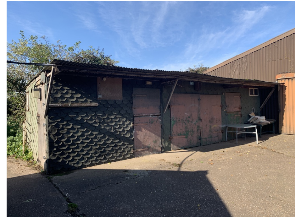
Front elevation showing Loose boxes and store.
