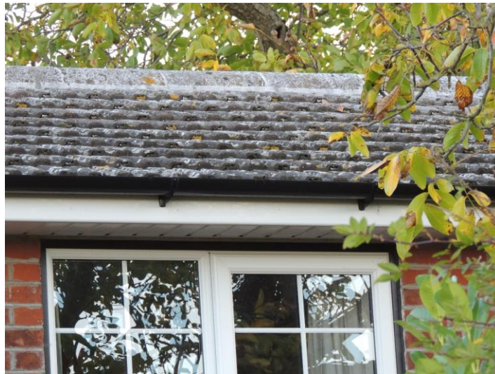
Photo 11: Showing tight seal to roof tiles
