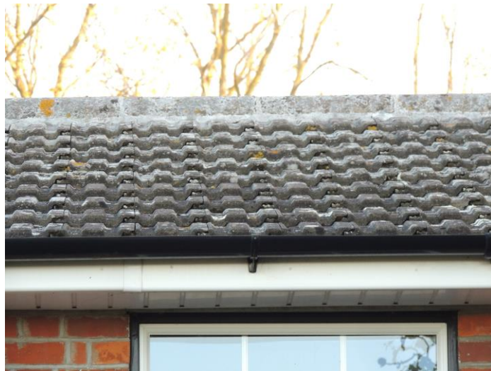
Photo 9: Showing tight seal to roof tiles
