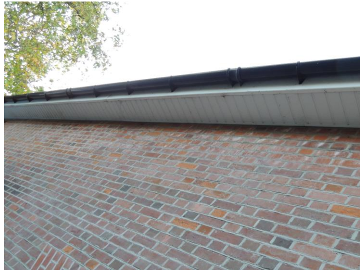
Photo 5: Showing tight seal to eaves
