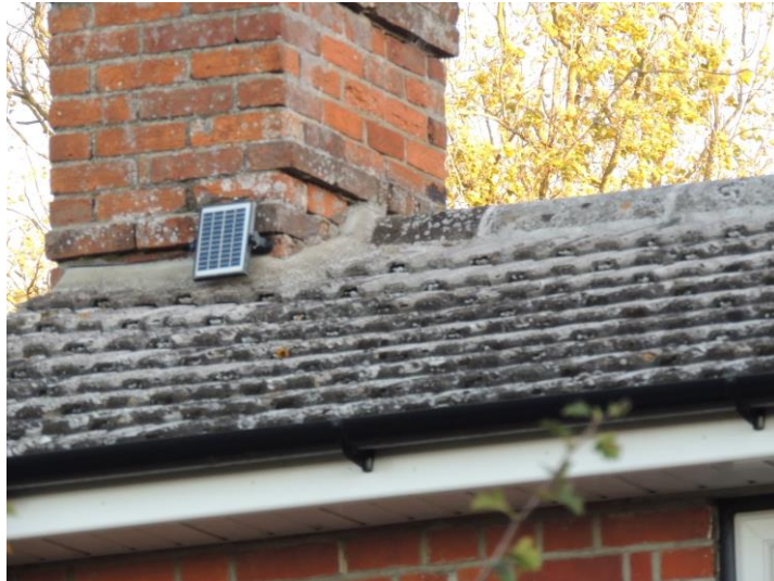
Photo 10: Showing tight seal to roof tiles and around chimney
