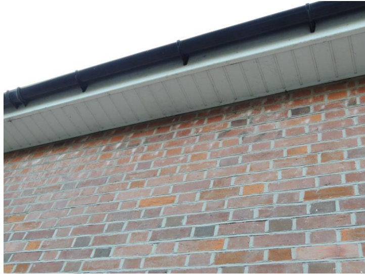
Photo 4: Showing tight seal to eaves
