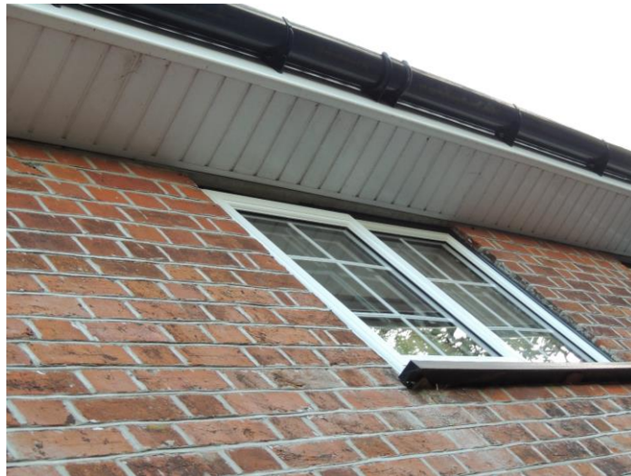
Photo 8: Showing tight seal to eaves on southern side
