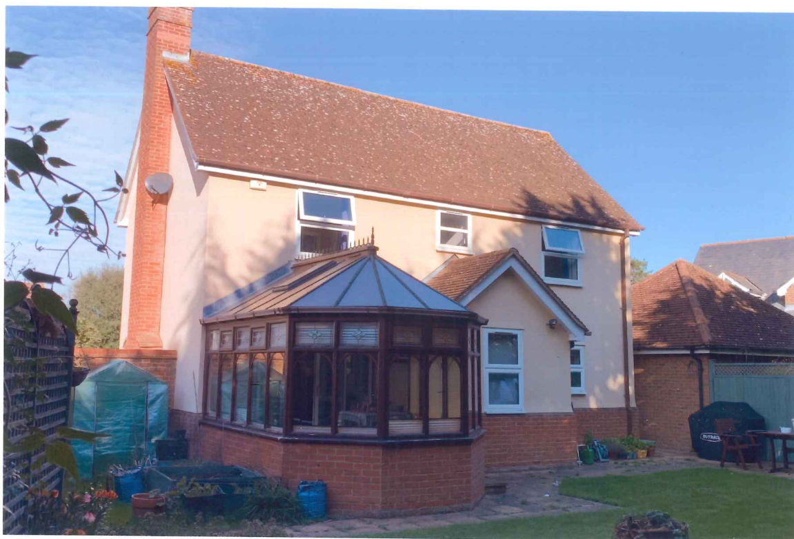
View of the Rear of the existing house from the garden.
