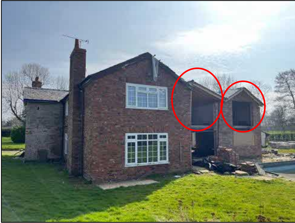
Photograph 4: A view of the rear of the building. Large entry points can clearly be seen (circled) creating ideal opening to a sheltered foraging space for bats.
