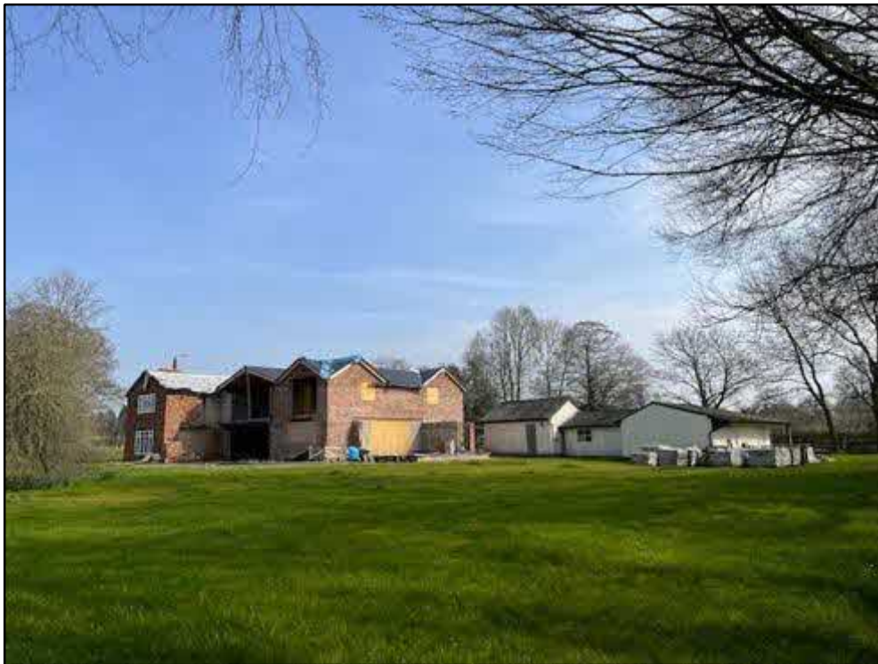
Photograph 5: A distant view from the south-westerly corner of the site. An adjacent garage building offers negligible bat roost and bird nesting potential. The stripped roof atop the main building can be seen.
