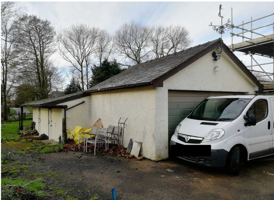
View south west from existing front driveway towards garage / stable block
