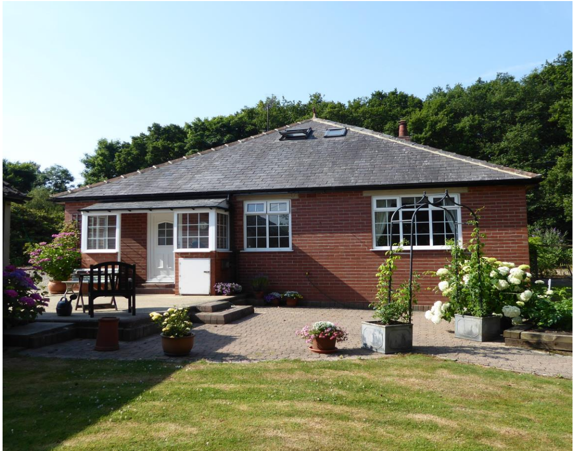
Photo 3 Rear, N E Elevation.
