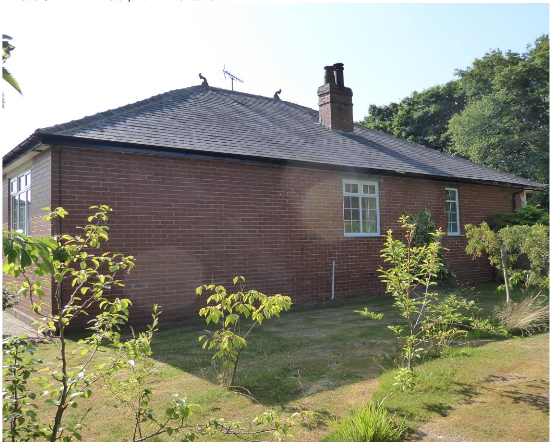
Photo. 4 Side, N W Elevation.
