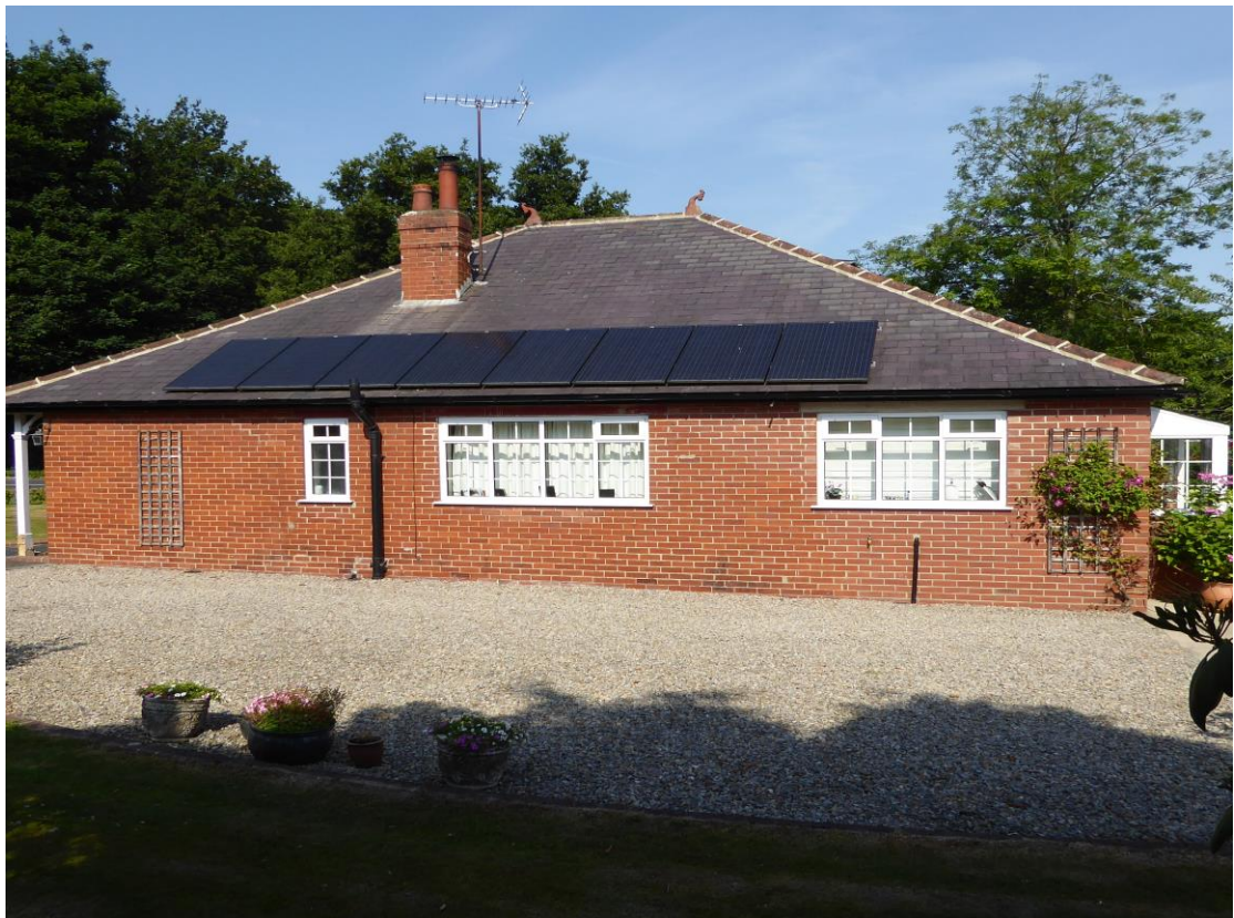
Photo. 2 Side, S E Elevation.
