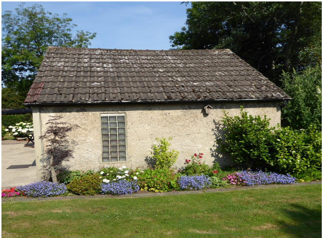
Photo. 2 Side, S E Elevation.
