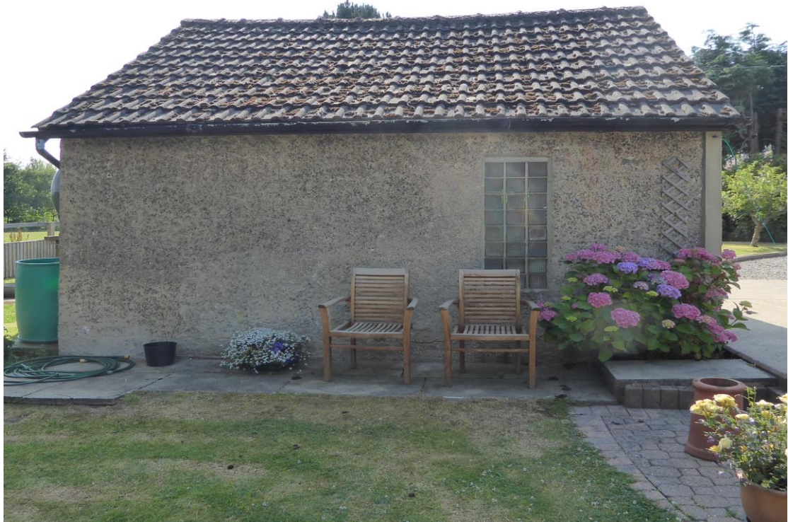
Photo. 4 Side, N W Elevation.
