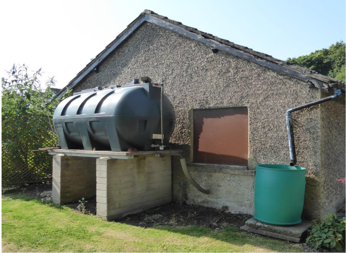
Photo 3 Rear, N E Elevation.
