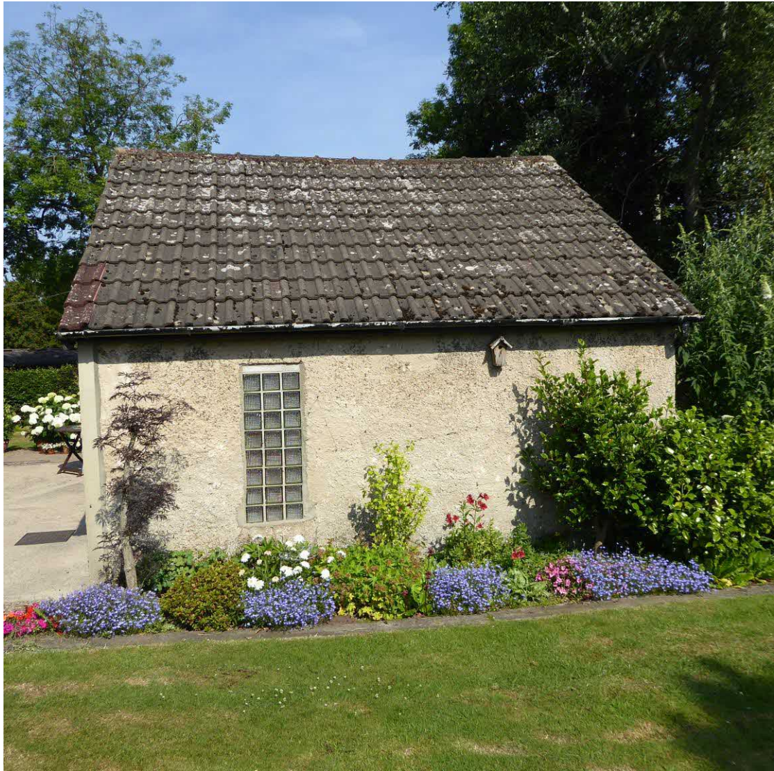
Photo. 2 Side; south east elevation.
