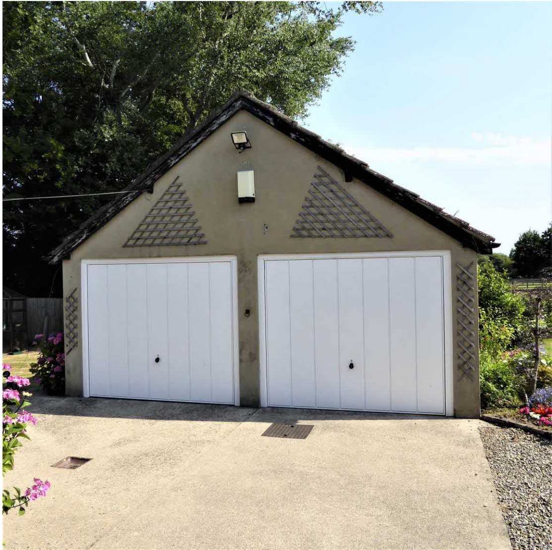
Photo. 1 Front; south west elevation.
