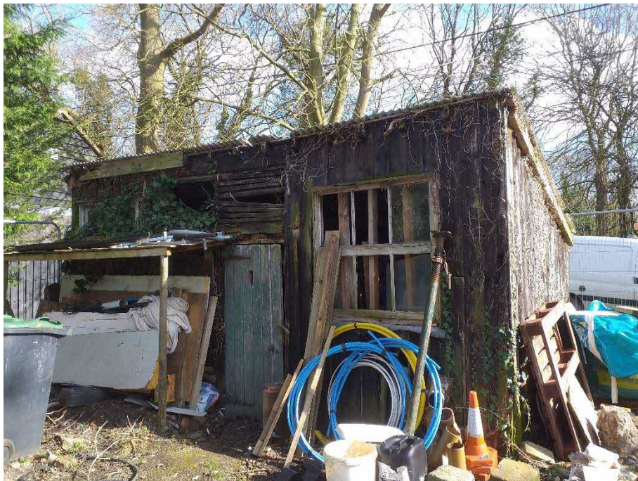
Shed in north eastern corner of site
