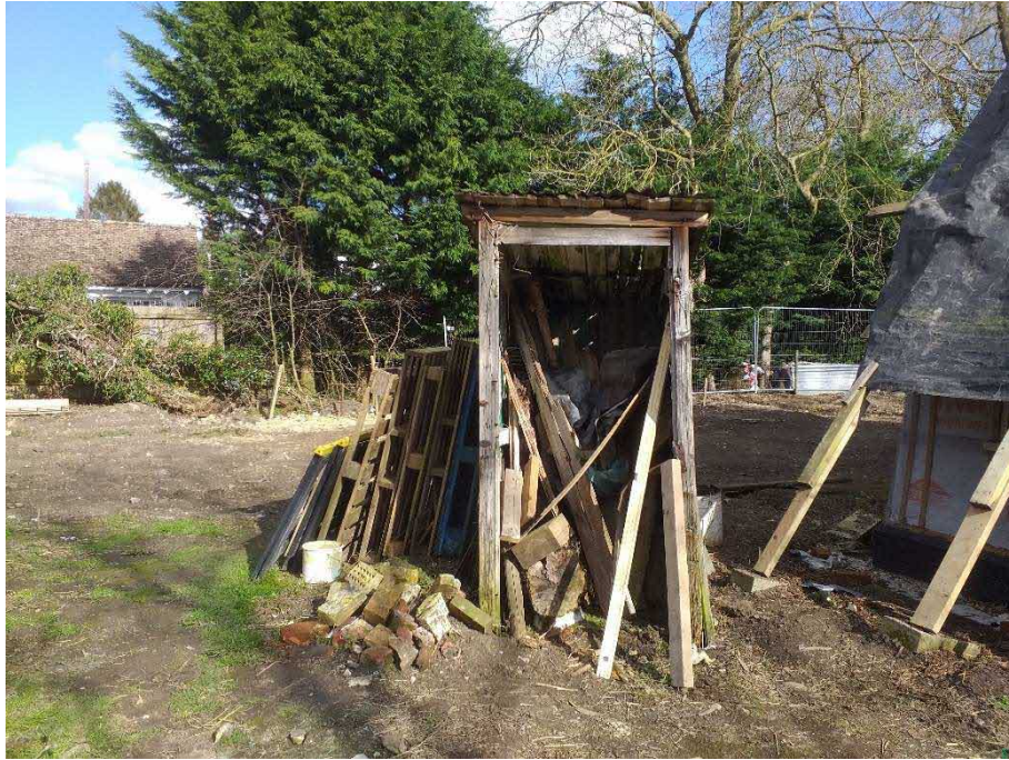
Former toilet building
