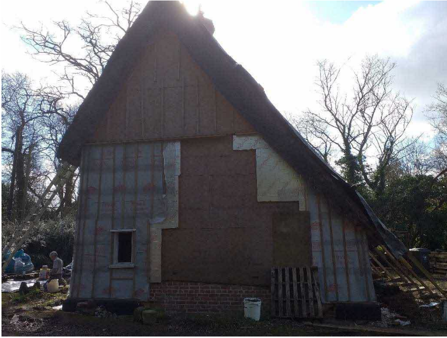
Northern elevation of cottage
