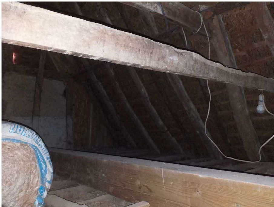
Roof void of loft. No evidence of bats
