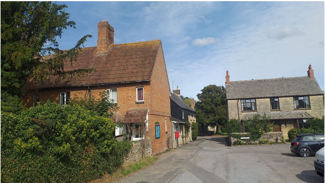
Photograph 4 of 15, 17 & 19 Church Street and 'The Square'
