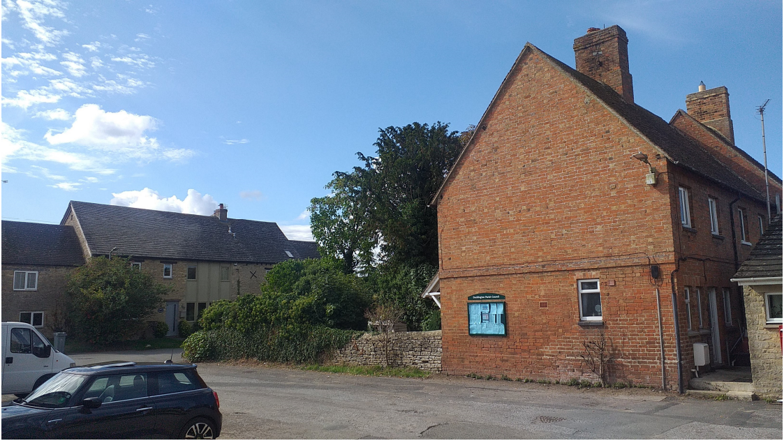
Photograph 1 of 15, 17 & 19 Church Street and 'The Square'
