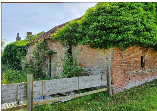
Figure 2: The barn northern and western aspect.
