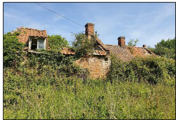
Figure 3: The barn – southern aspect.
