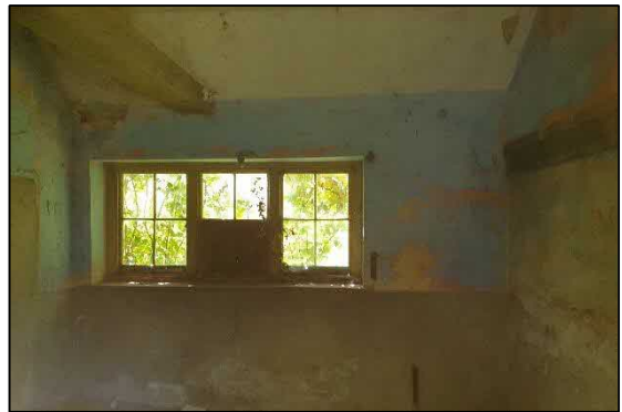
Figure 6: Room 4 – boarded ceiling leaving a low roof void.
