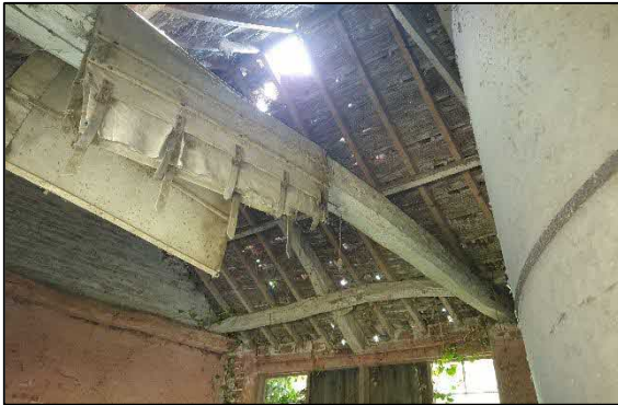
Figure 4: Internal view of western-most room
