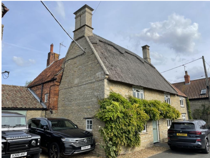
The photograph above shows the pantile garage roof to the left hand side which is to be extended vertically on the same footprint
