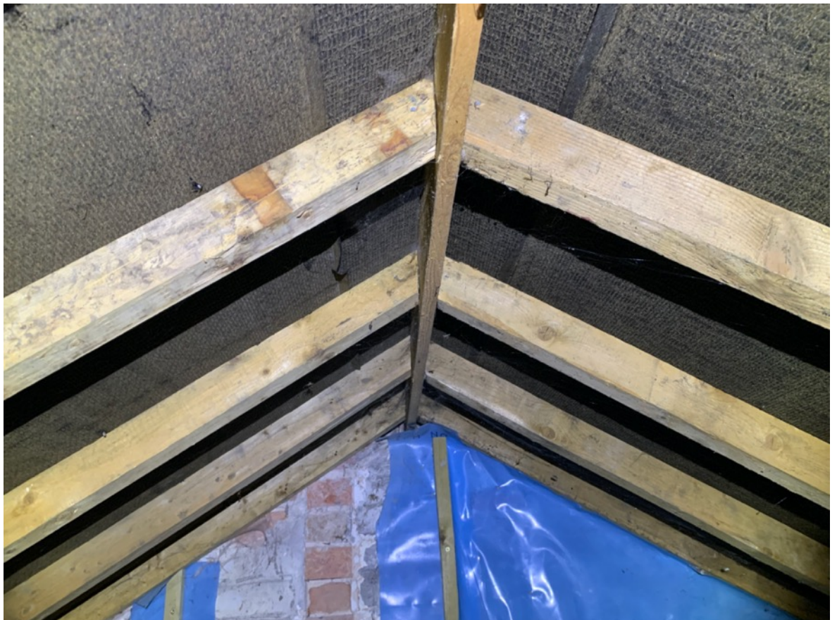
Photograph 3. Interior of Outbuilding roof void
