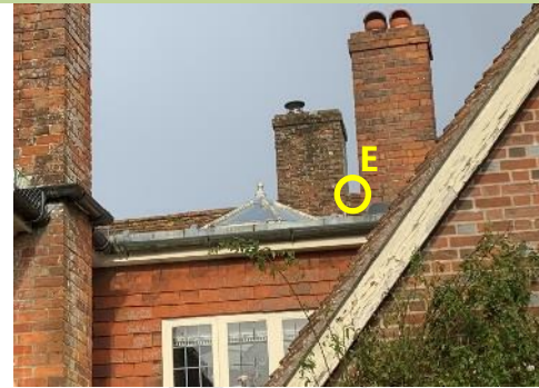
Bat Emergence point E
